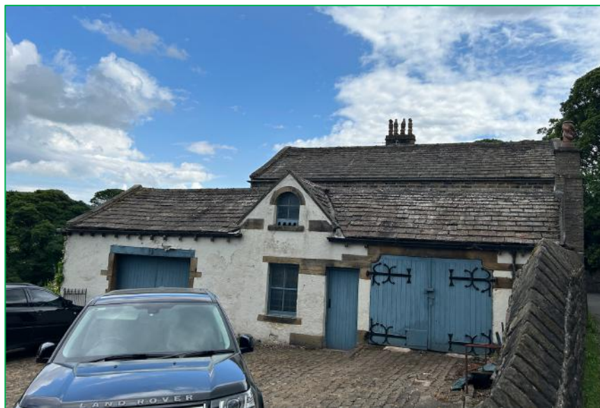
The northwest elevation of Netherfield House Barn
