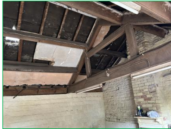
The interior of the garage
