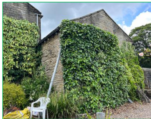
The northeast elevation of the workshop and garage
