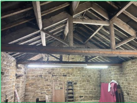
The upper floor of the large barn
