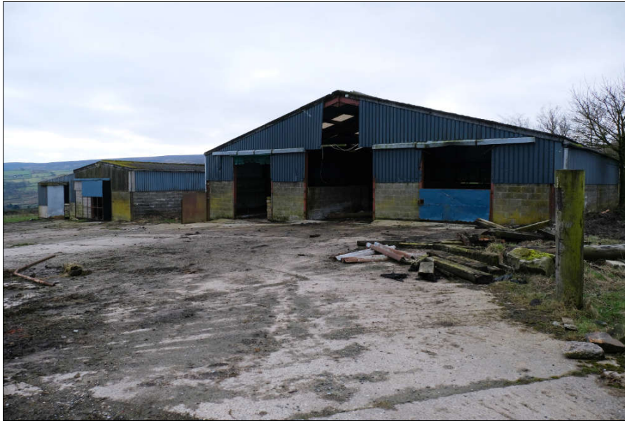
Building 1 (RHS) and building 2 (LHS) – exterior view. The buildings are accessible to barn owls and other bird species
