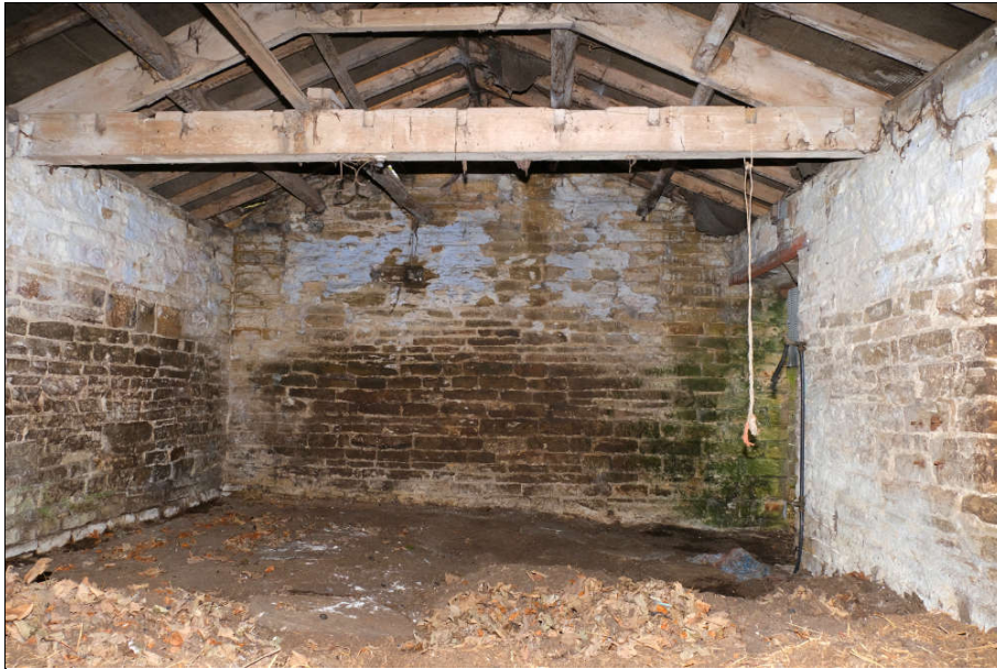
Interior of building 5, showing a range of perching points for barn owls, and also a lack of nesting resources (platforms).
