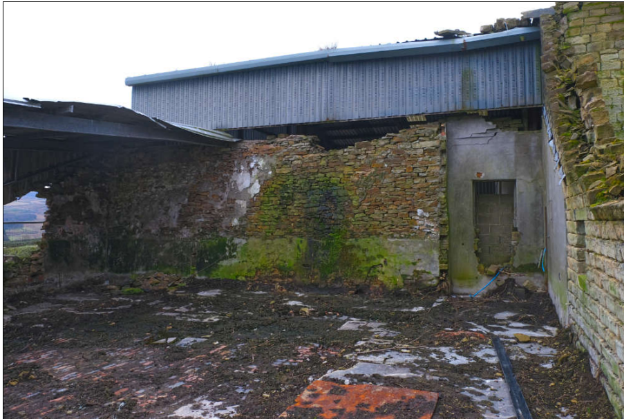
Building 4 – no roof present. This part of the site offers almost negligible potential for use by barn owls for roosting and no potential for barn owl nesting.
