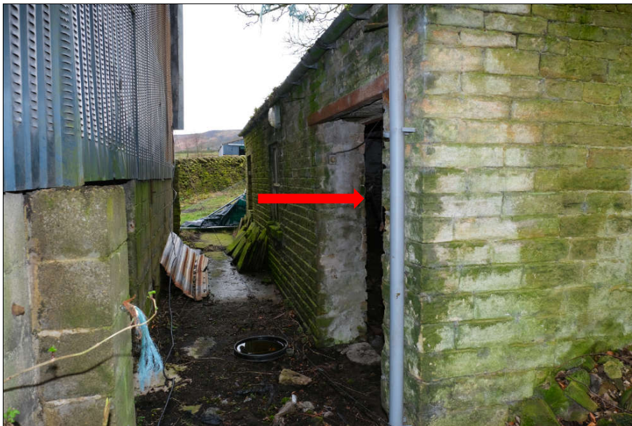
Building 5, showing the likely main access point for the barn owl – an open door to the south elevation. This doorway lies close to building 3 (agricultural barn) and is in a sheltered position, helping to minimise light spillage and draughts.
