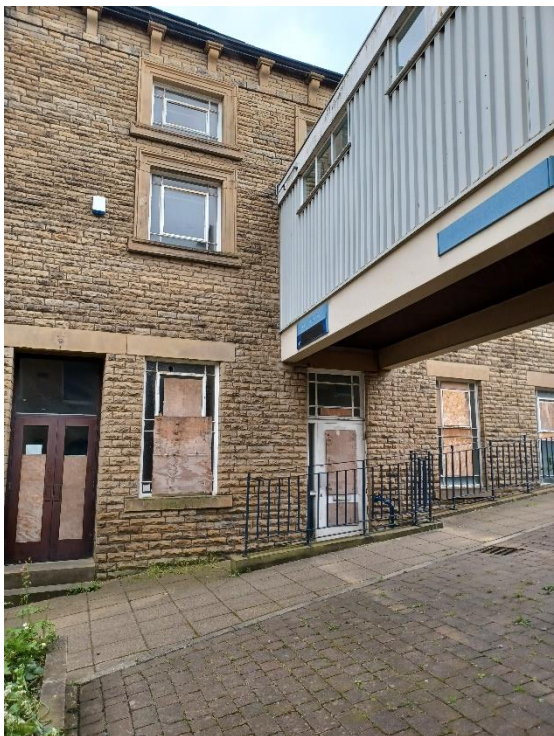
Photo 2: Link bridge connected through former original fenestration opening on Brunswick Building Elevation
