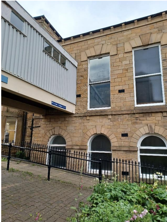
Photo 2: Link bridge connected through former original fenestration opening on Batley Town Hall Elevation
