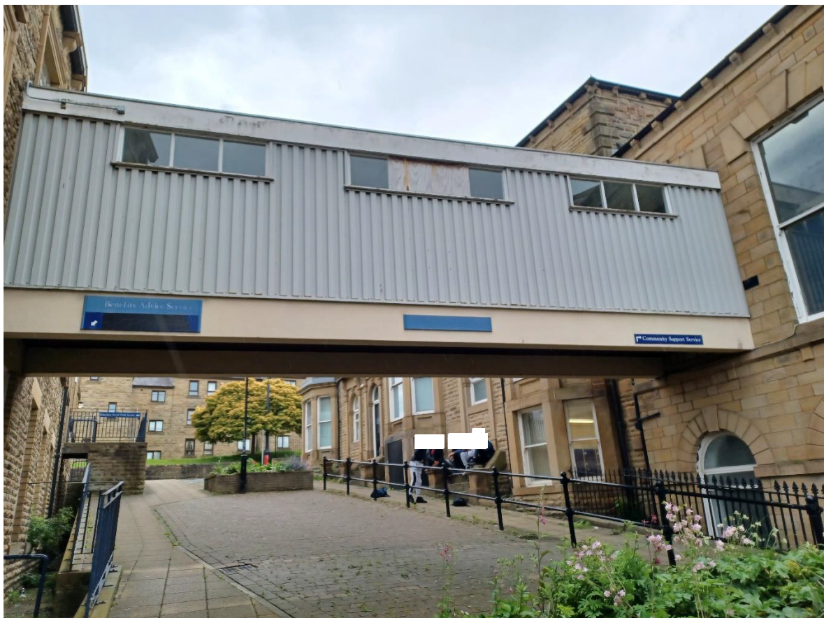
Photo 1: Link bridge exterior view
