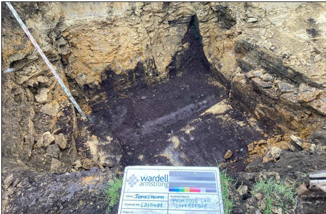
Figure 5: Image showing the aperture of mine entry 419424-014 at a depth of 2.2m bgl and surrounded by sandstone bedrock.
