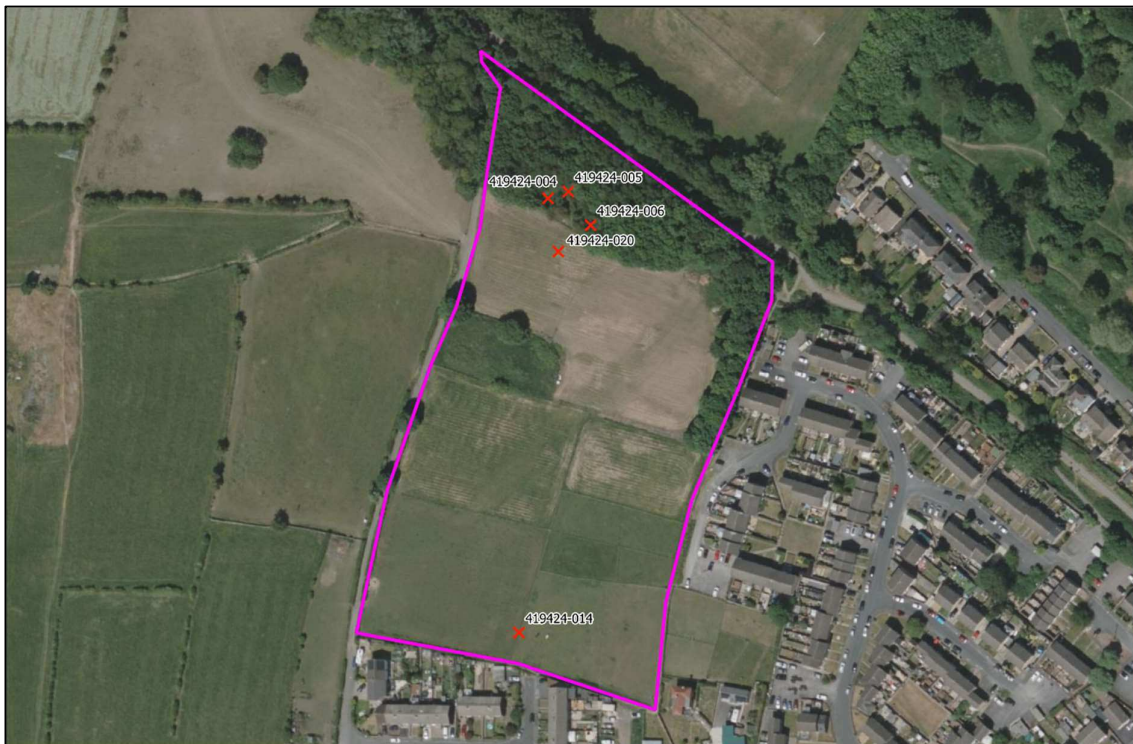
Figure 4: Image showing the updated mine entry locations based on CA data and recent investigations. 4
