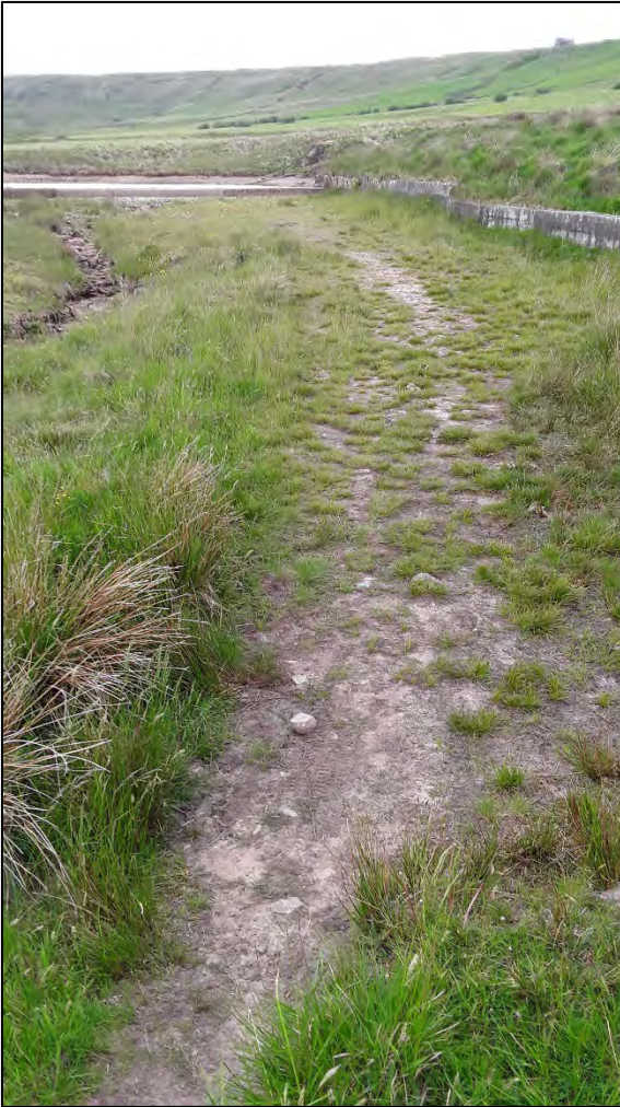
T1 looking west towards the reservoir, close to the western end
