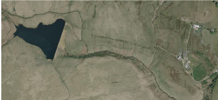
Figure 1 - Aerial View of Reservoir
