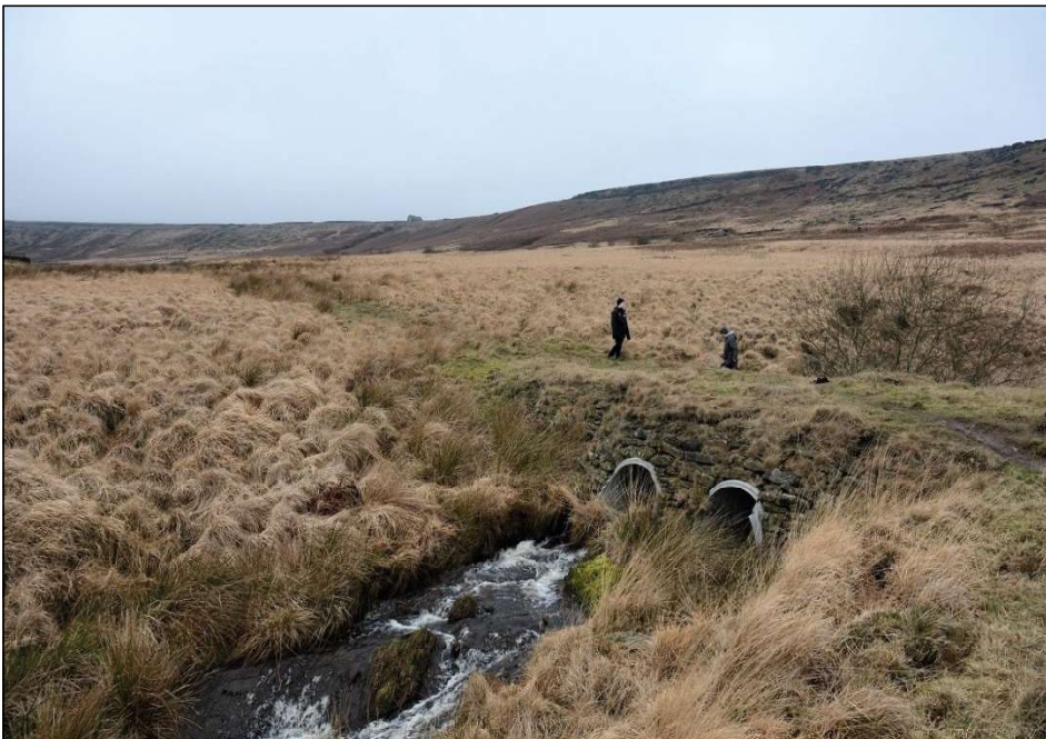
Plate 8. Temporary access track bridge built in the 1990s, looking north-west
