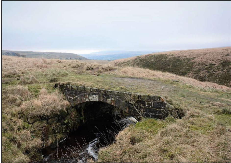
Plate 5. The 19th-century bridge close to the reservoir dam, looking east
