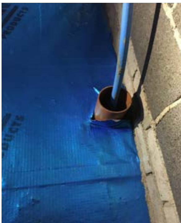
A small aperture is cut for the service.
