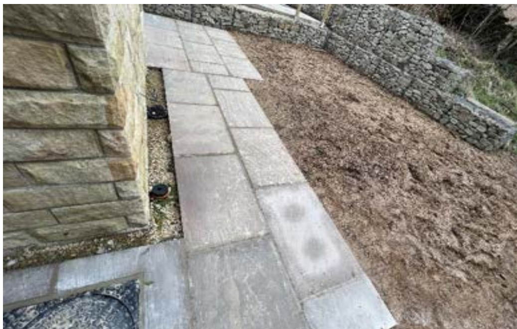
Finished hard paving to the rear.
