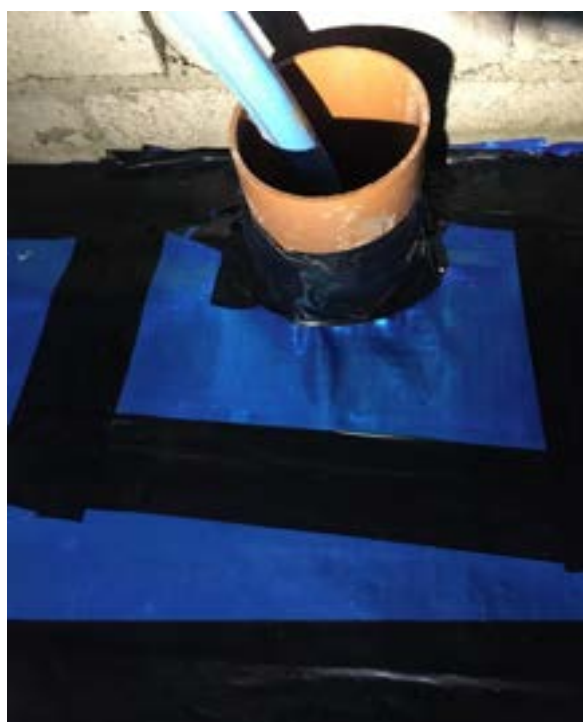
The seams between the layers and the interface with the service pipe are then taped over with single sided tape.
