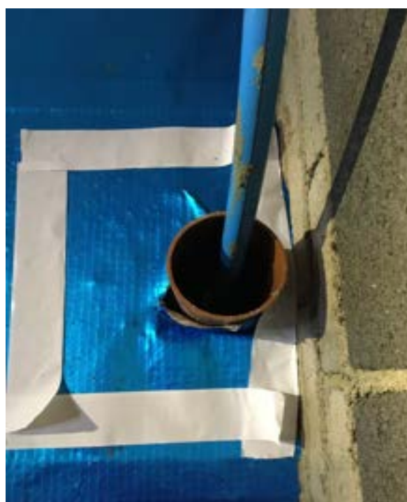
double sided mastic sealing tape is placed around the aperture.
