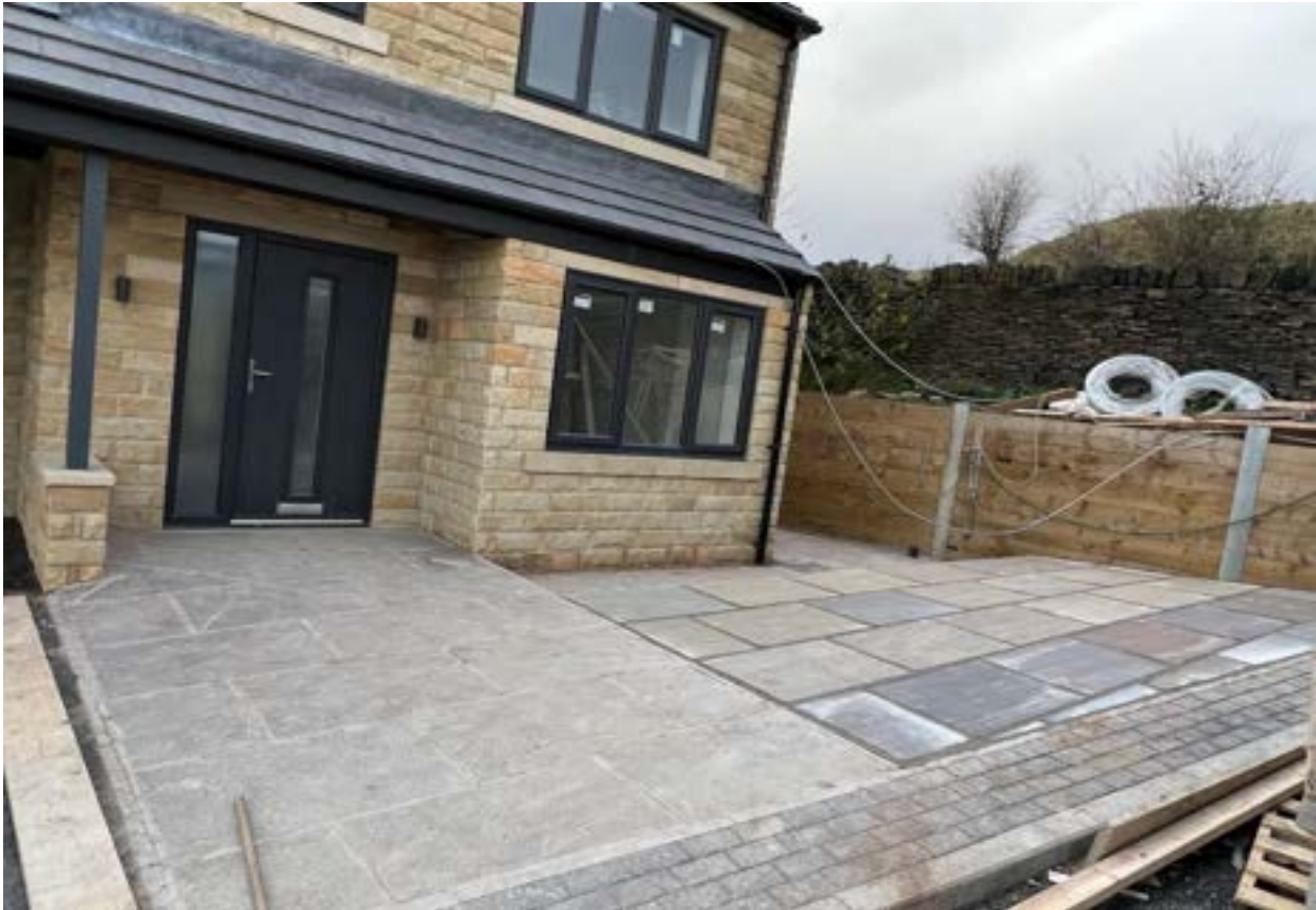
FRONT HARD PAVING ON COMPLETION
