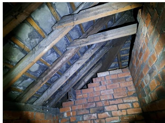
Photograph 19 Showing a section of roof void of B1
