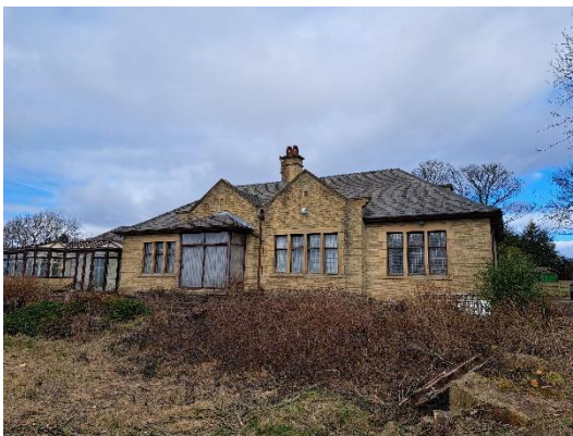
Photograph 16: Showing the southern elevation of B1
