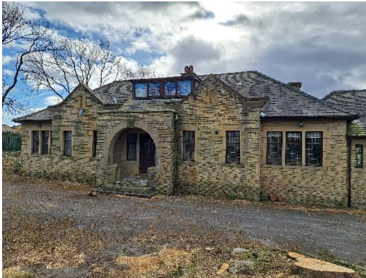
Photograph 14: Showing the northern elevation of B1
