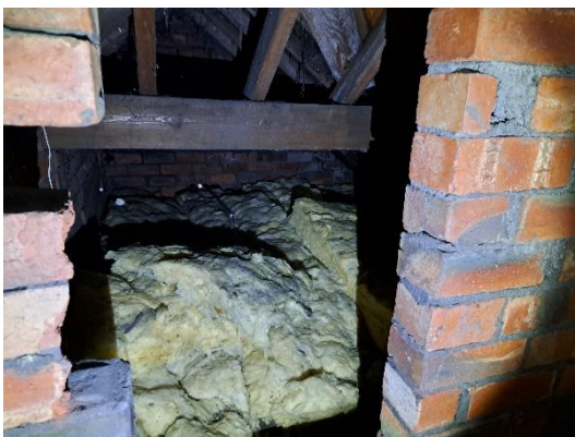
Photograph 18: Showing a section of roof void of B1
