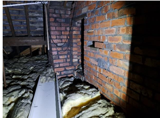
Photograph 21: Showing a section of roof void of B1
