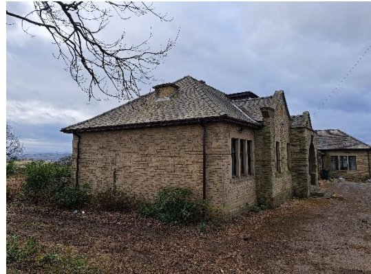
Photograph 15: Showing the eastern elevation of B1
