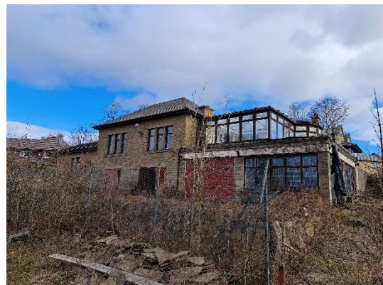
Photograph 17: Showing a section of the southern and western elevations of B1
