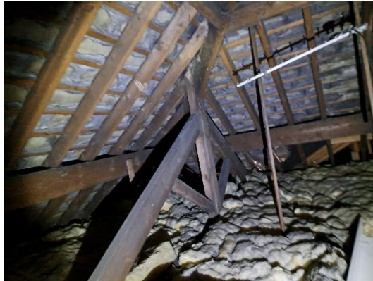
Photograph 20: Showing a section of roof void of B1
