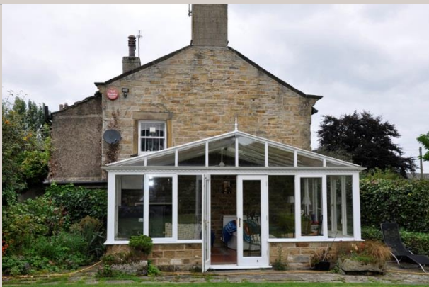
Figure 13: Modern conservatory added to gable end with ground floor window converted to a door to link this to the house
