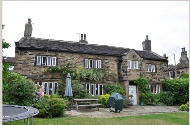
Figure 12: East front as observed from the private garden. Retains original window pattern of three, four and five light mullions. The two storey porch was probably an addition since it has larger stone blocks and a break either side of the drip course. The high door surround is more commonly found in 18 th century buildings in this area
