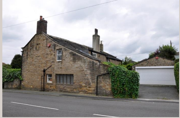
Figure 10: Street facing elevation with rebuilt service extension to form a kitchen diner, entrance lobby and bathroom over (compare to figure 6 ). Note survival of two older mullion windows (one window blocked). Modern garage
