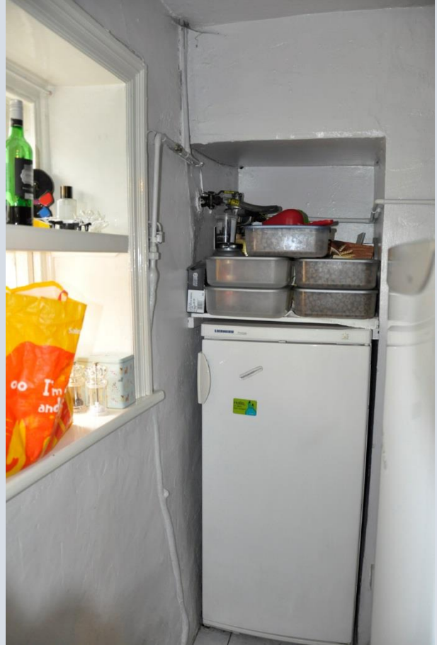
Figure 16: Recess marks blocked door opening from pantry to study, ground floor
