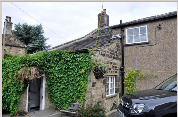
Figure 14: Rendered rear elevation with altered windows and part rebuilt service extension that forms kitchen with bathroom over
