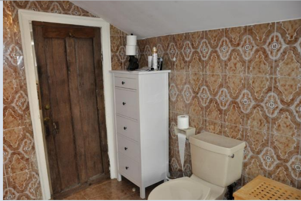
Figure 19: Modern bathroom with c.1800 panelled door
