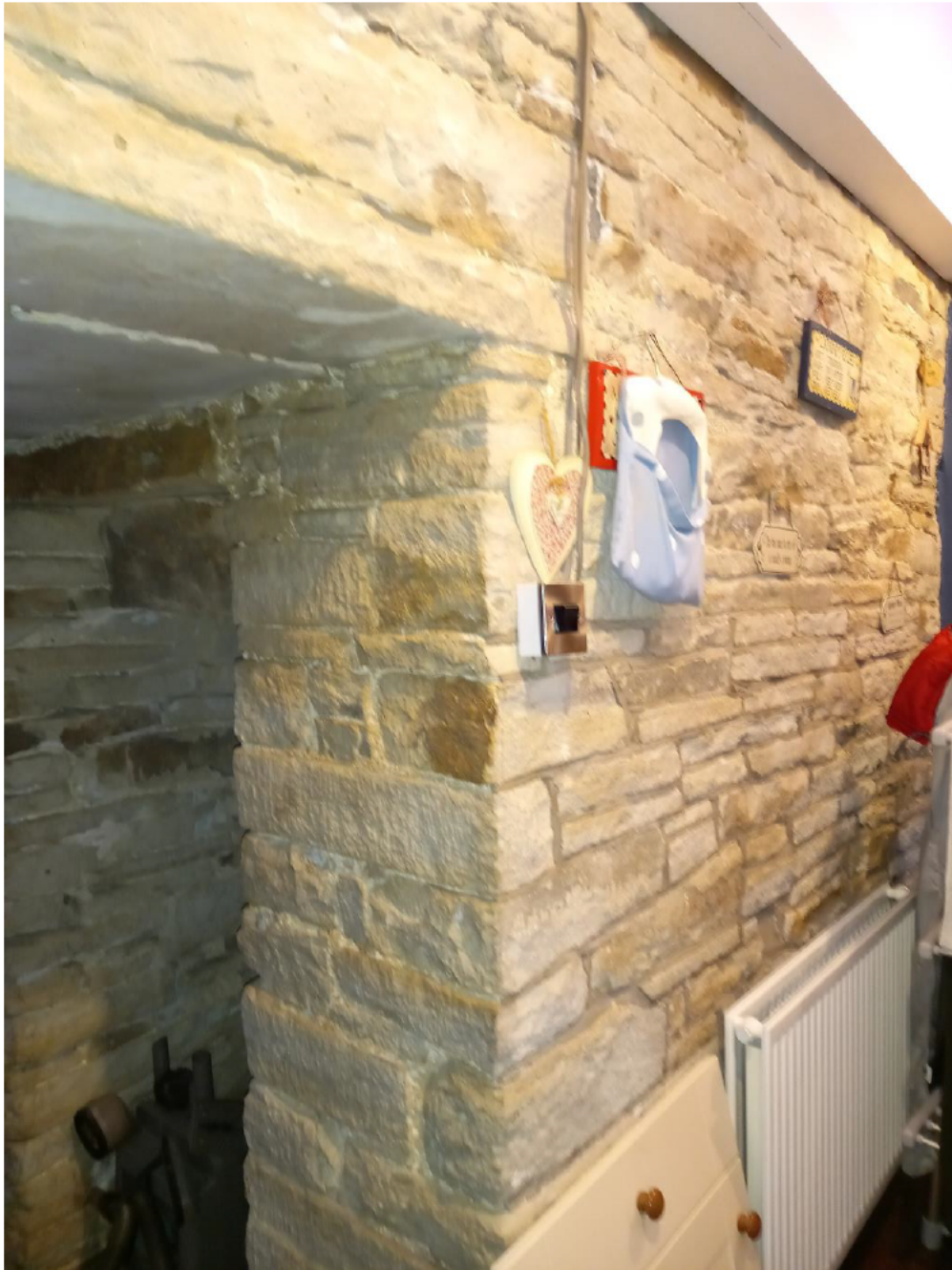
Utility with stonework exposed and retained internally
