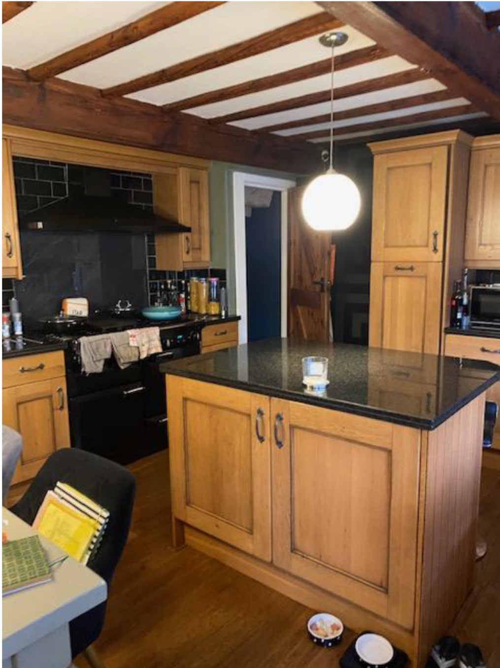
Internal kitchen view with floor joists exposed internally
