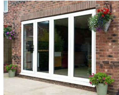
Fig 5.13 - White uPVC bifolding doors
