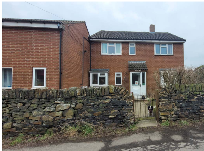
Fig 3.3: View of the front elevation to the existing dwelling.
