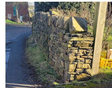
Fig 5.16 - Existing stone boundary wall to be partially demolished and re-built.
