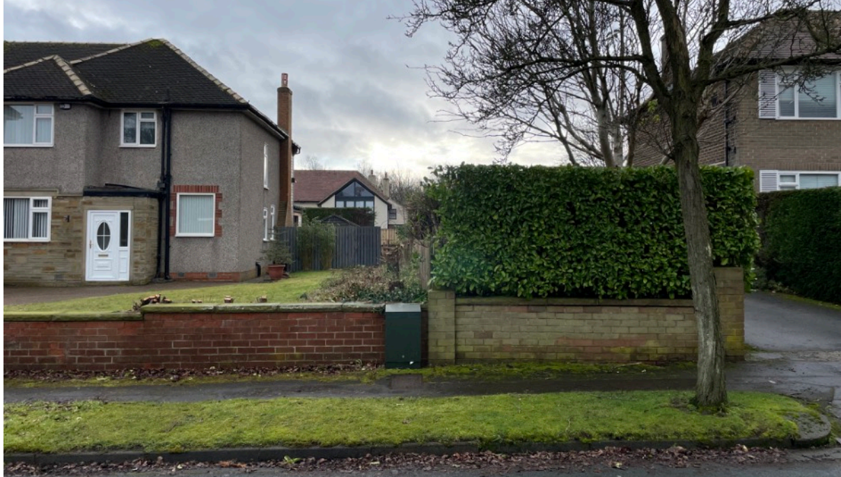
View of North elevation.
