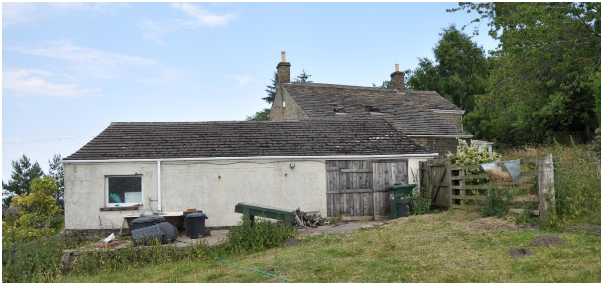
3. Photograph of the rear taken from the west.
