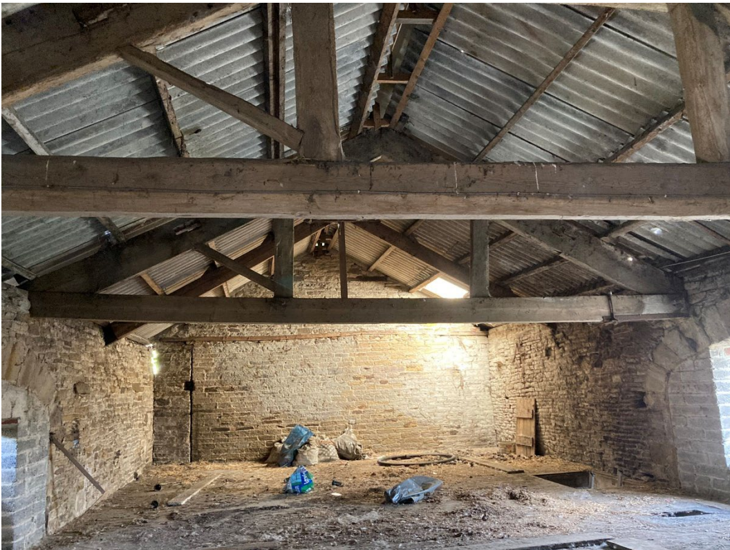
Photo 7. Building 7 interior – looking to north gable
