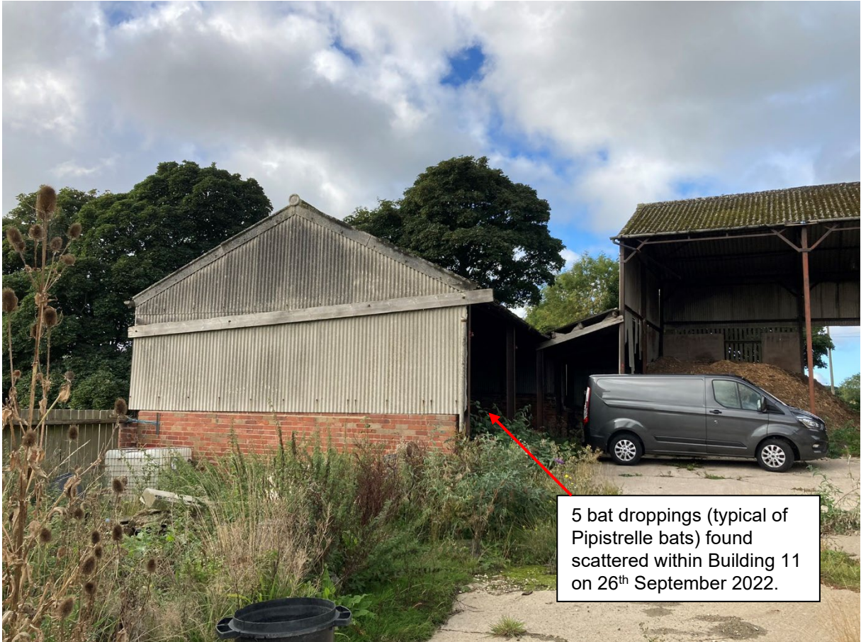
Photo 3. Looking west to Buildings 10 (left) and Building 11 (right)
