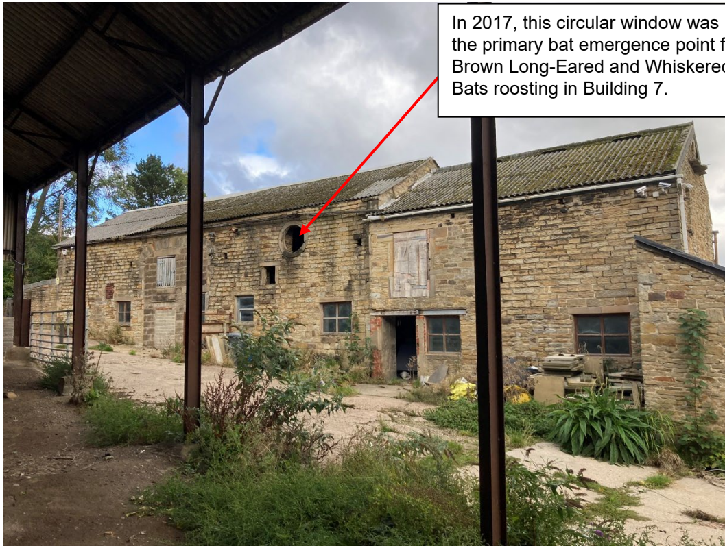
Photo 1. Buildings 7 and 5 – west elevations (taken from within Building 10)
