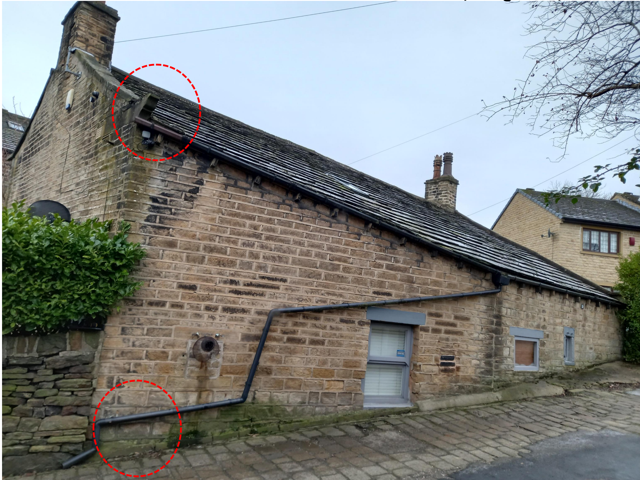
Gaps on the parapet coping but no sign of bats roosting or bats droppings
