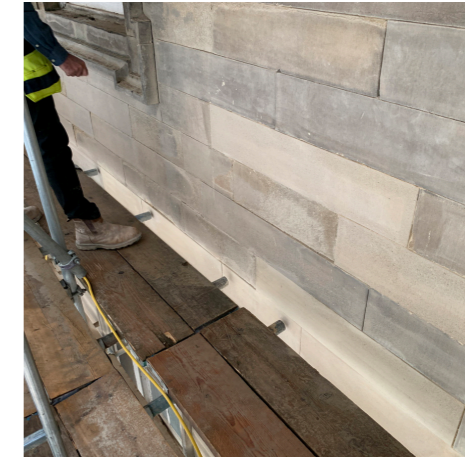
PHOTO A : Localised Masonry Repair
