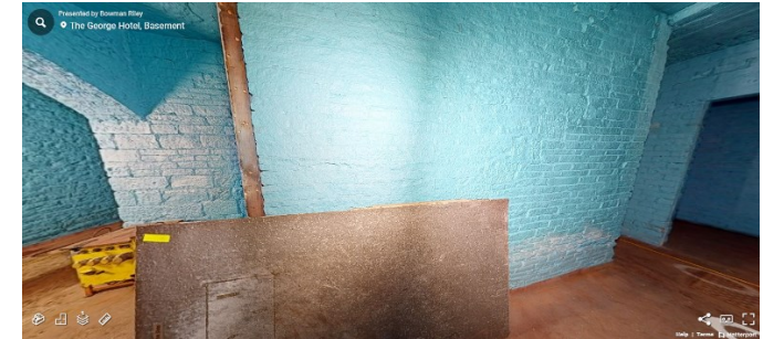
Evidence of former openings (top) and stairs (bottom).
