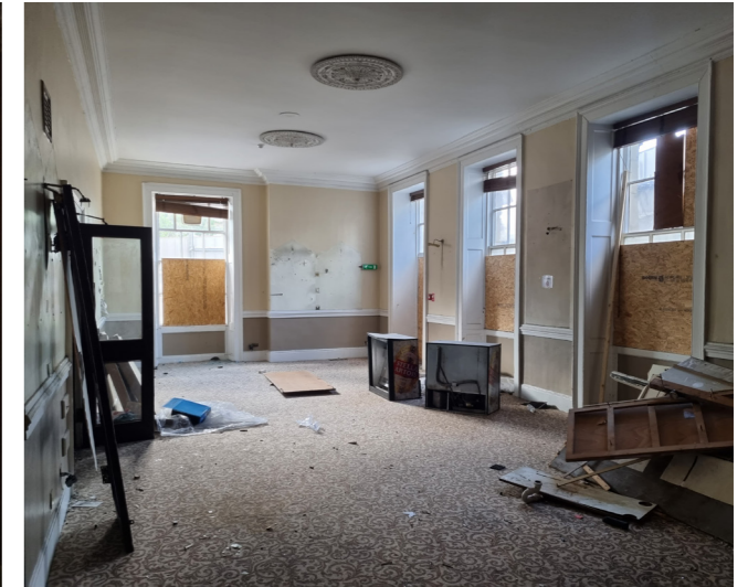
PHOTO 3 Ground Floor view of the former Bar & Event space
