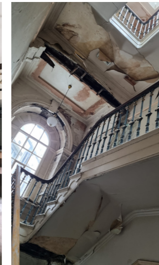
PHOTO 7 GF view of main staircase.
