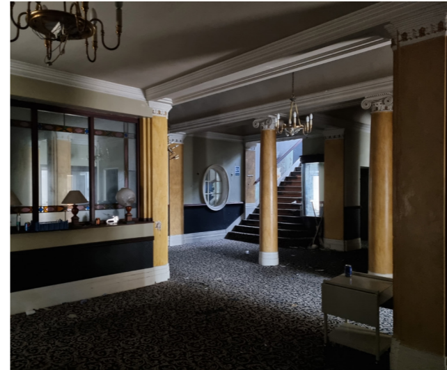
PHOTO 2 Ground Floor view of the entrance space and main staircase.
