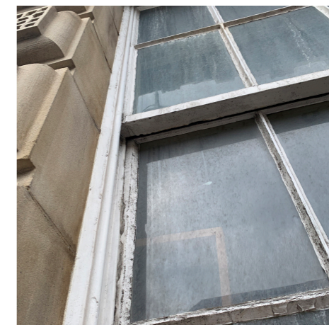
PHOTO C : Phase 2 existing window condition
