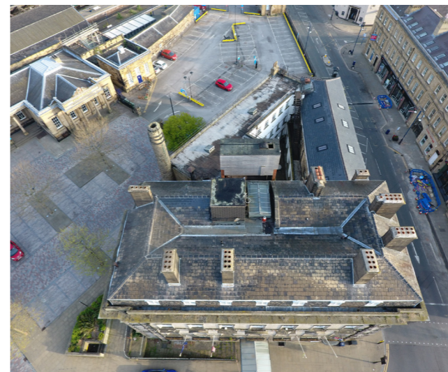
PHOTO 11 Drone view facing Block A from the south.
