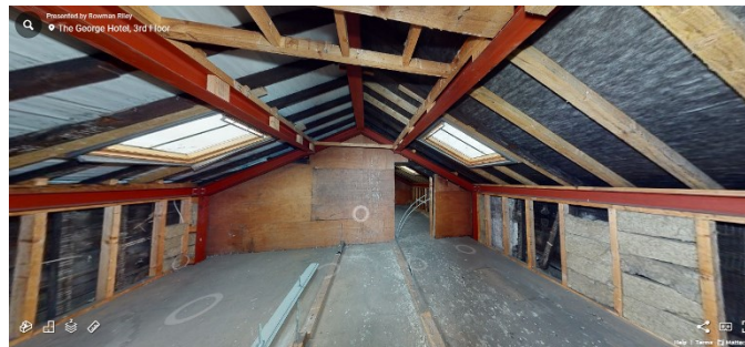
Steel frame to the third floor of Block C.
