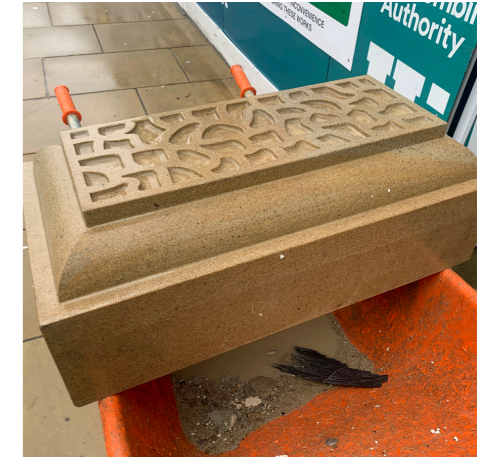
PHOTO B : Masonry repair of complete unit
