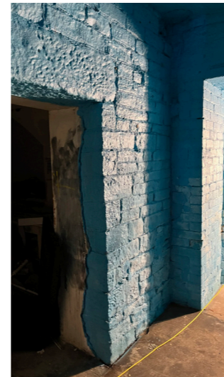
PHOTO 5 Basement view of circulation.
