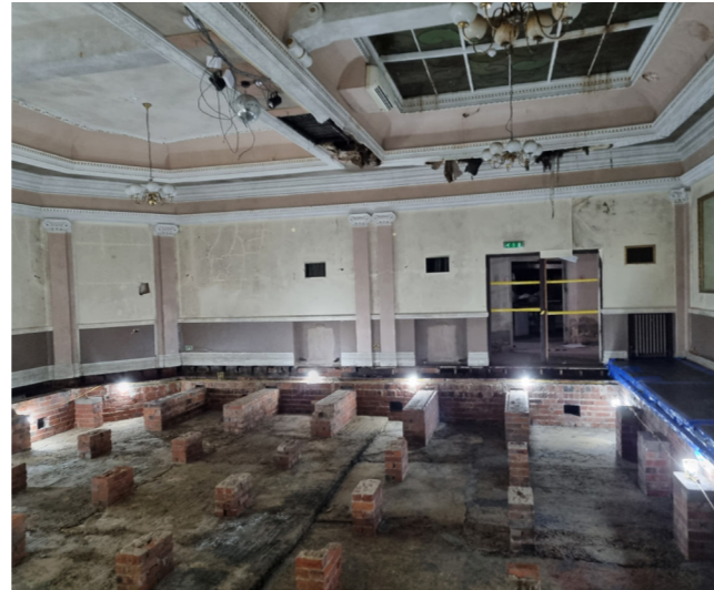
PHOTO 1 Ground Floor view of the former Ballroom.
