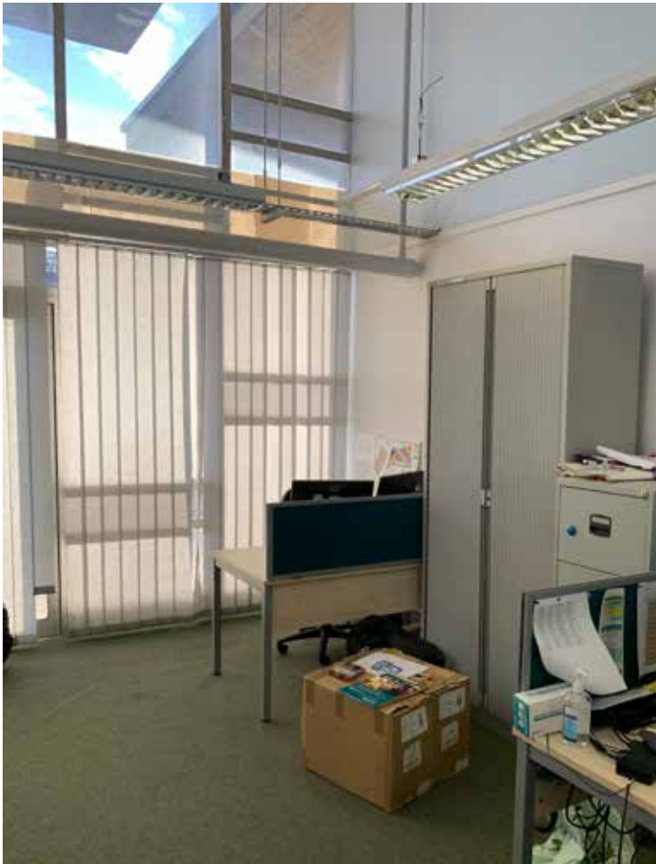
FF-22 - Partition formed abutting the curtain glazing and rising as a solid element to the concrete soffit
