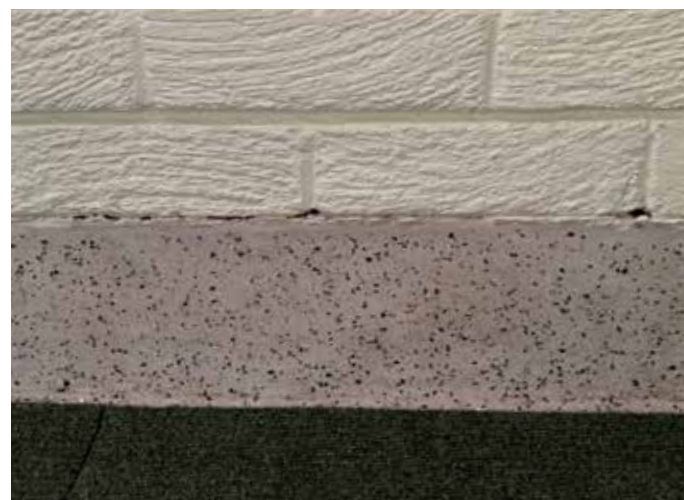
Above: FF-05 - Original lift button Below: FF-05 - Concrete / terrazzo plinth to the wall
