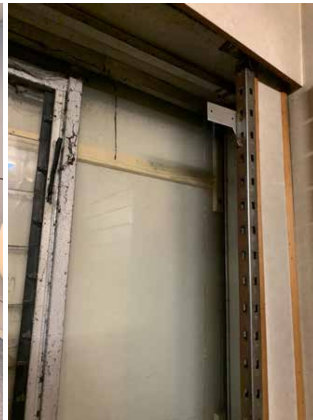
GF-MH-168a - Original south-facing glazing overboarded
