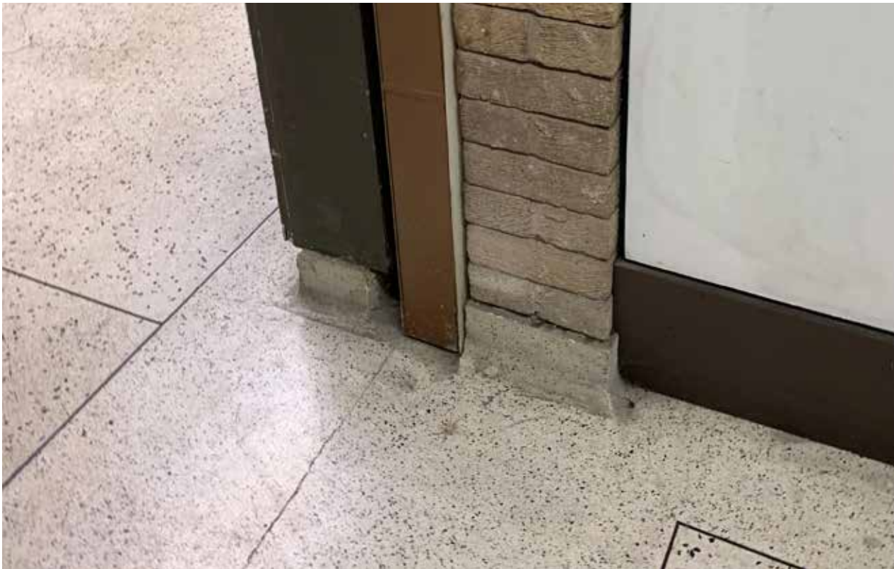
FF-06 - Terrazzo floor with coved skirting and pocket fire door set behind a metal panelled wall
