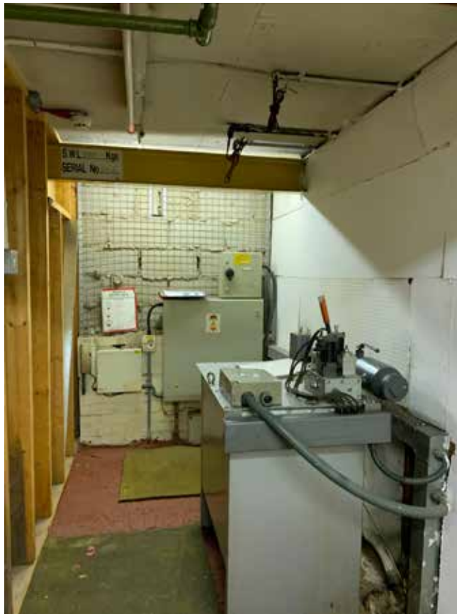
Plant room with pump set for hydraulic lift
