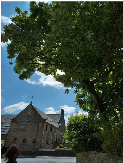
Photo 5: T30 and T33 from north east.
