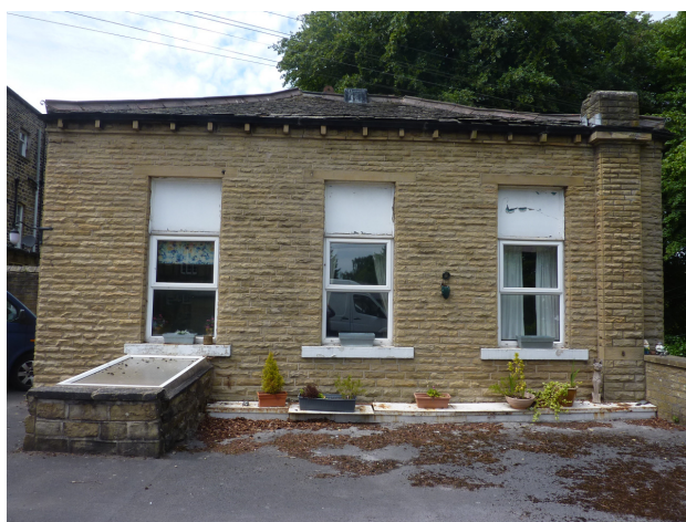
View of the south east facing elevation
