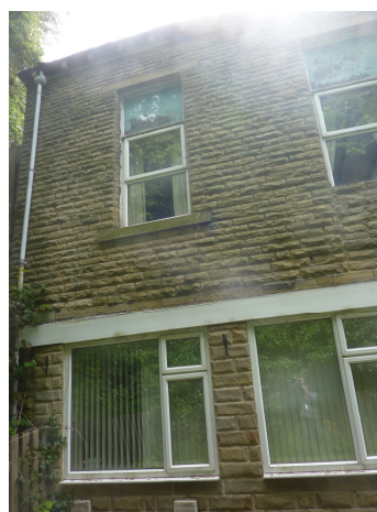
Part of the north east facing elevation from the lower level
