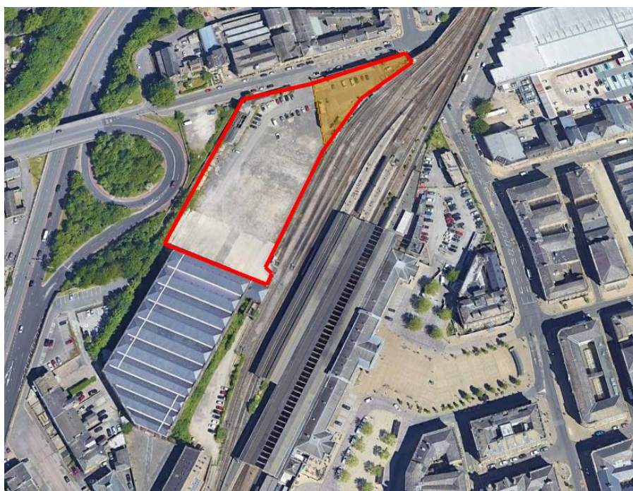
Insert 5-1 Aerial photo of the former goods storage area at Huddersfield Station with the area identified for watching brief highlighted in orange
