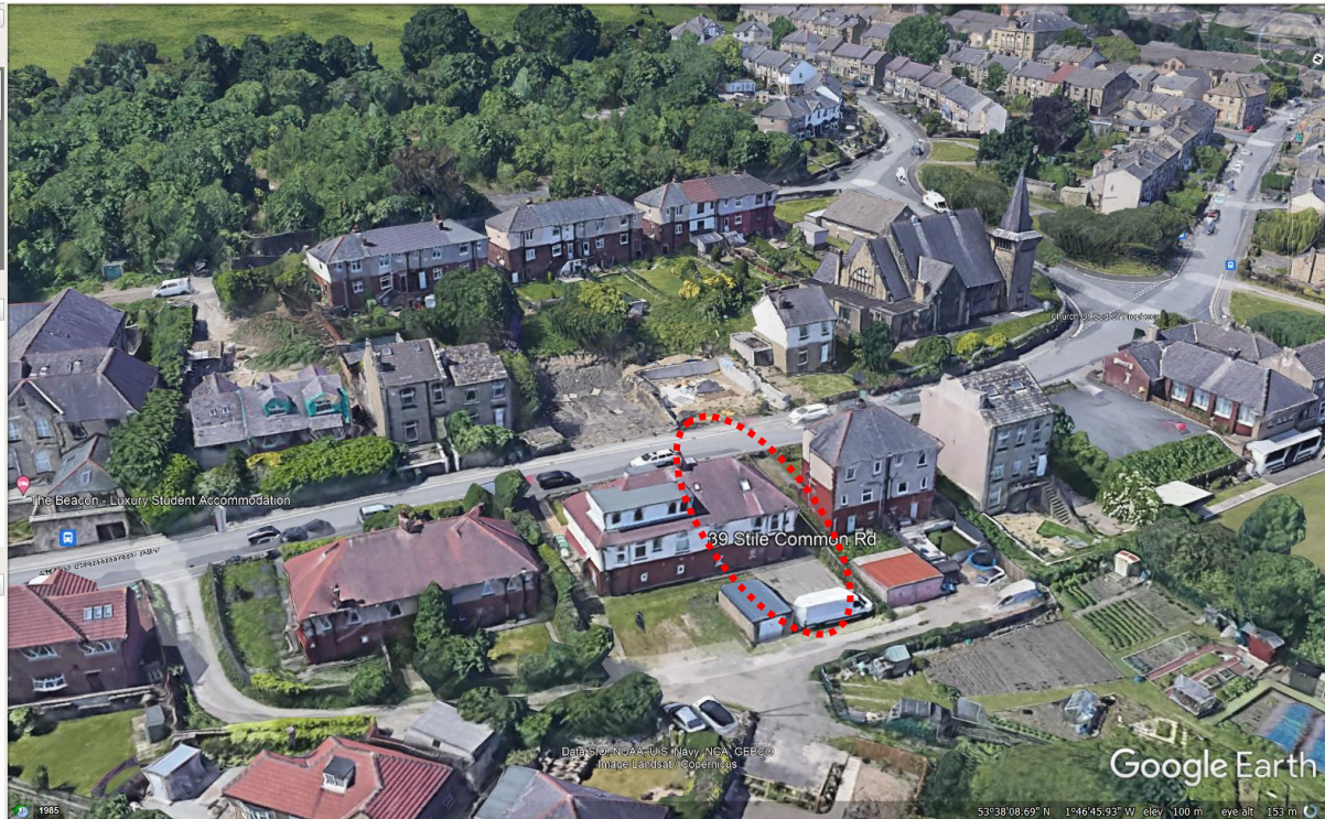
Rear aerial view
