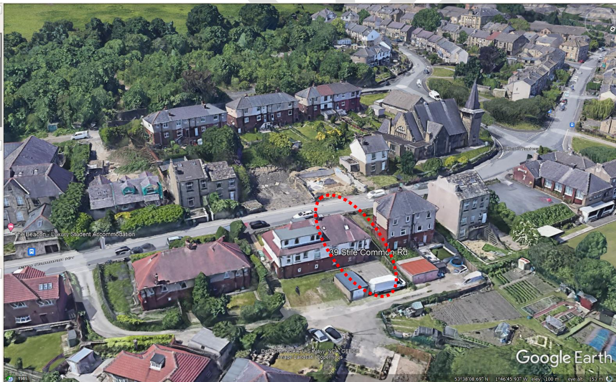
Rear aerial view
