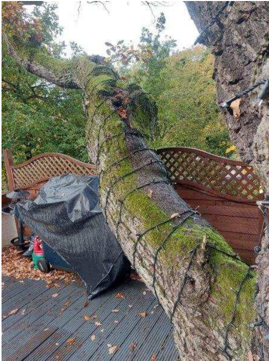
Photo 5: View along the low horizontal primary limb extending to the south-west side, with decay (brown rot) visible on the upper side of a main section.
