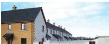
Social Housing Installation Co. Louth, Ireland
