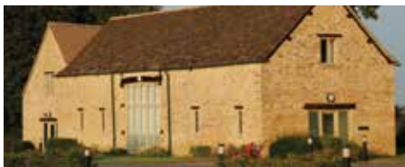
Barn Conversion Wing, England
