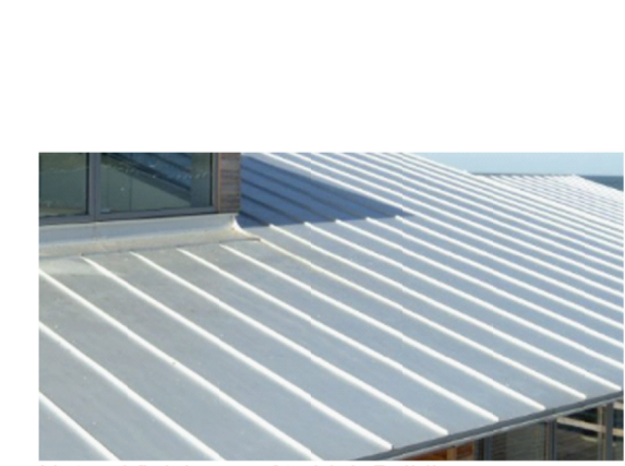
Natural finish – roof to Link Building
