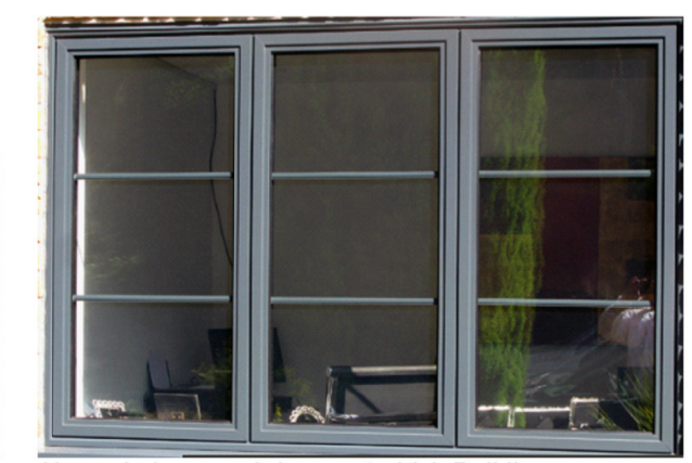
New windows and doors – to Link Building
