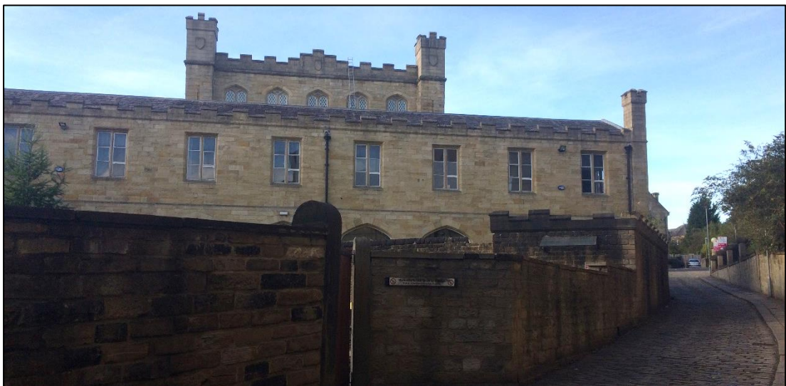
Plate 4. Boundary wall from Highfields Lane
