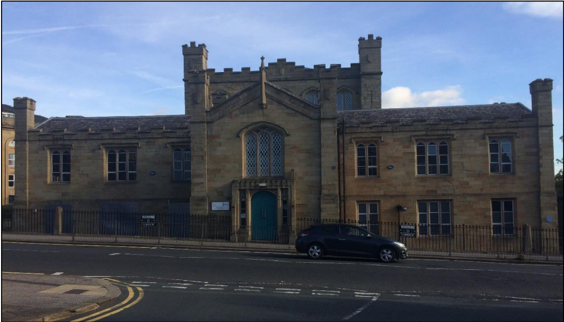
Plate 6. Elevation facing Highfields Lane
