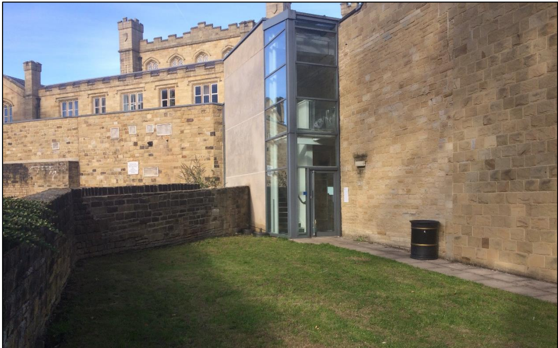
Plate 3. Amenity grass and boundary wall
