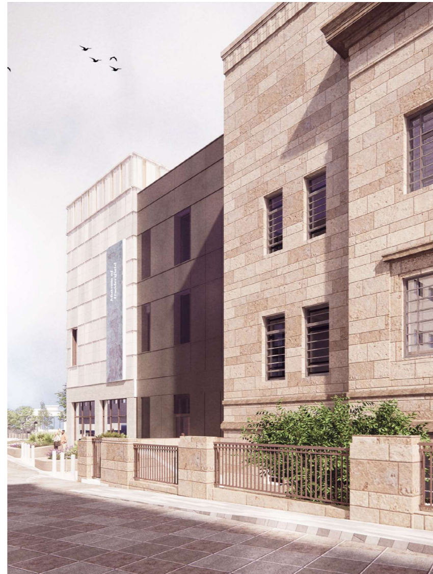
Proposed Amendment 1 Reduced mullions to accentuate horizontals & perforate panels in front of windows/ false windows. Signage zone shown indicatively on new stone extension.
