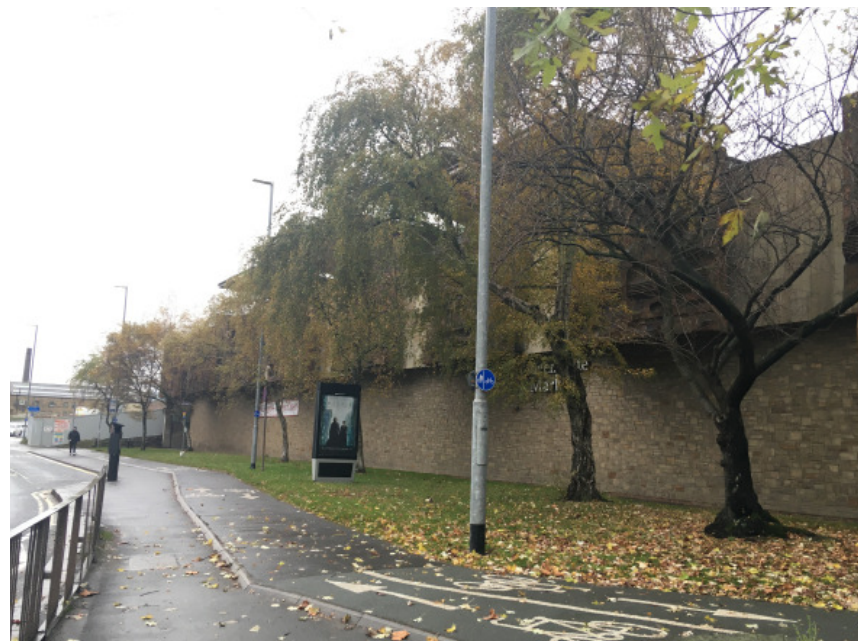
Fig.6.5.9 Existing Birch and Plane trees along Queensgate approaching life expectancy and block views of ceramic friezes on the market hall
