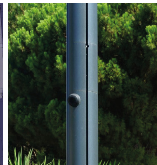
Fig.19.1.3 CCTV cameras discreetly contained within lighting columns
