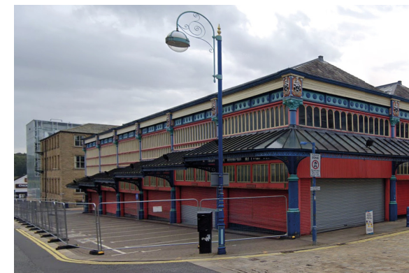
Fig.13.2.5 Victorian replica steel decorative lamp columns outside outdoor market
