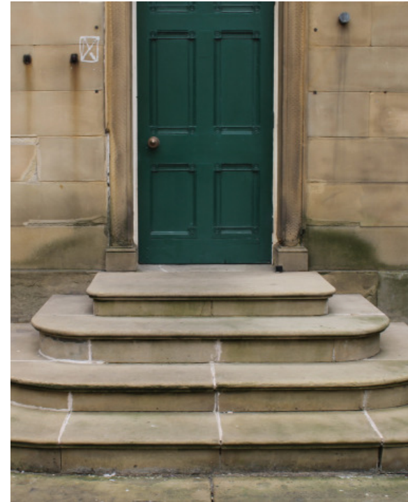
Fig.13.1.1 Locally sourced sawn Yorkstone stairs at Lawrence Batley Theatre
