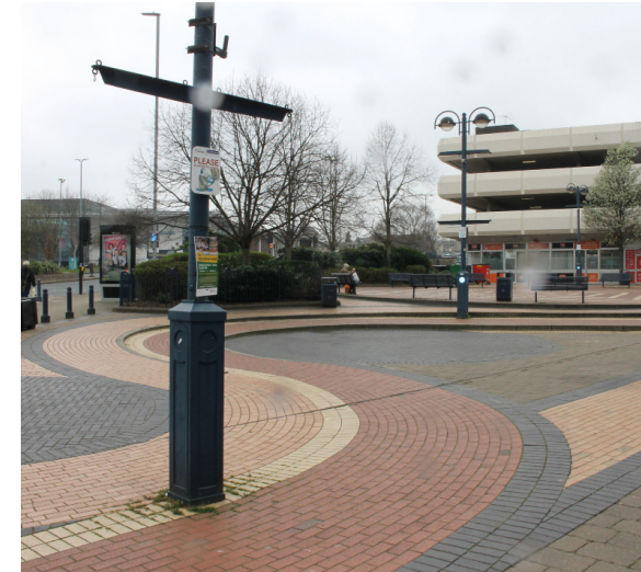
Fig.13.2.2 Multiple tones of brick used to create surface pattern by the bus station
