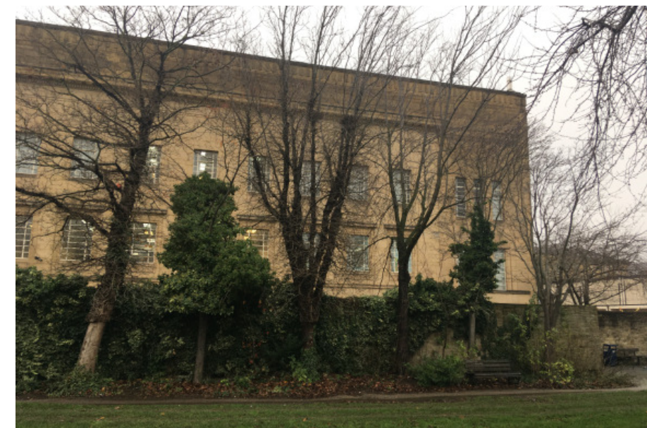
Fig.14.6 Existing trees along Huddersfield Library
