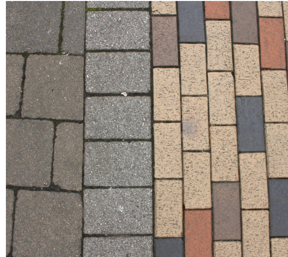
Fig.13.2.1 Concrete block and brick pavers used in a variety of arrangements
