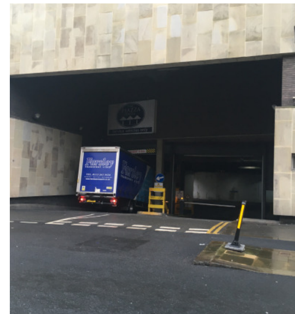
Fig.6.5.11 Basement tunnel access from Queen Street dominates the streetscape
