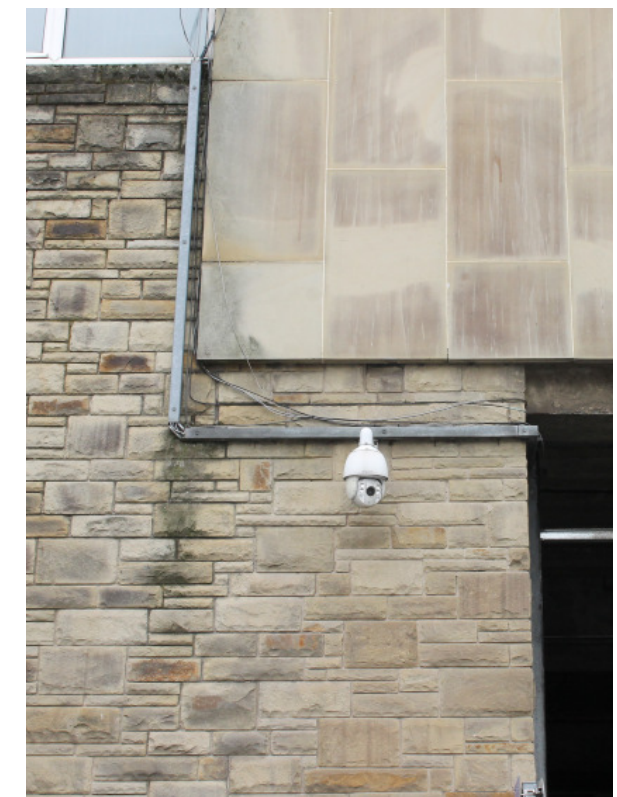
Fig.13.1.6 Sandstone cladding on existing Piazza shopping centre on Queen Street; sawn and split faced
