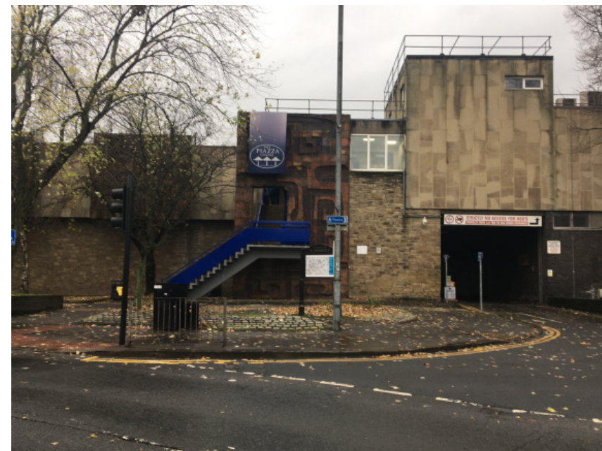
Fig.6.5.10 Pedestrian steps and tunnel entrance from Queensgate is unwelcoming and lack of accessible route
