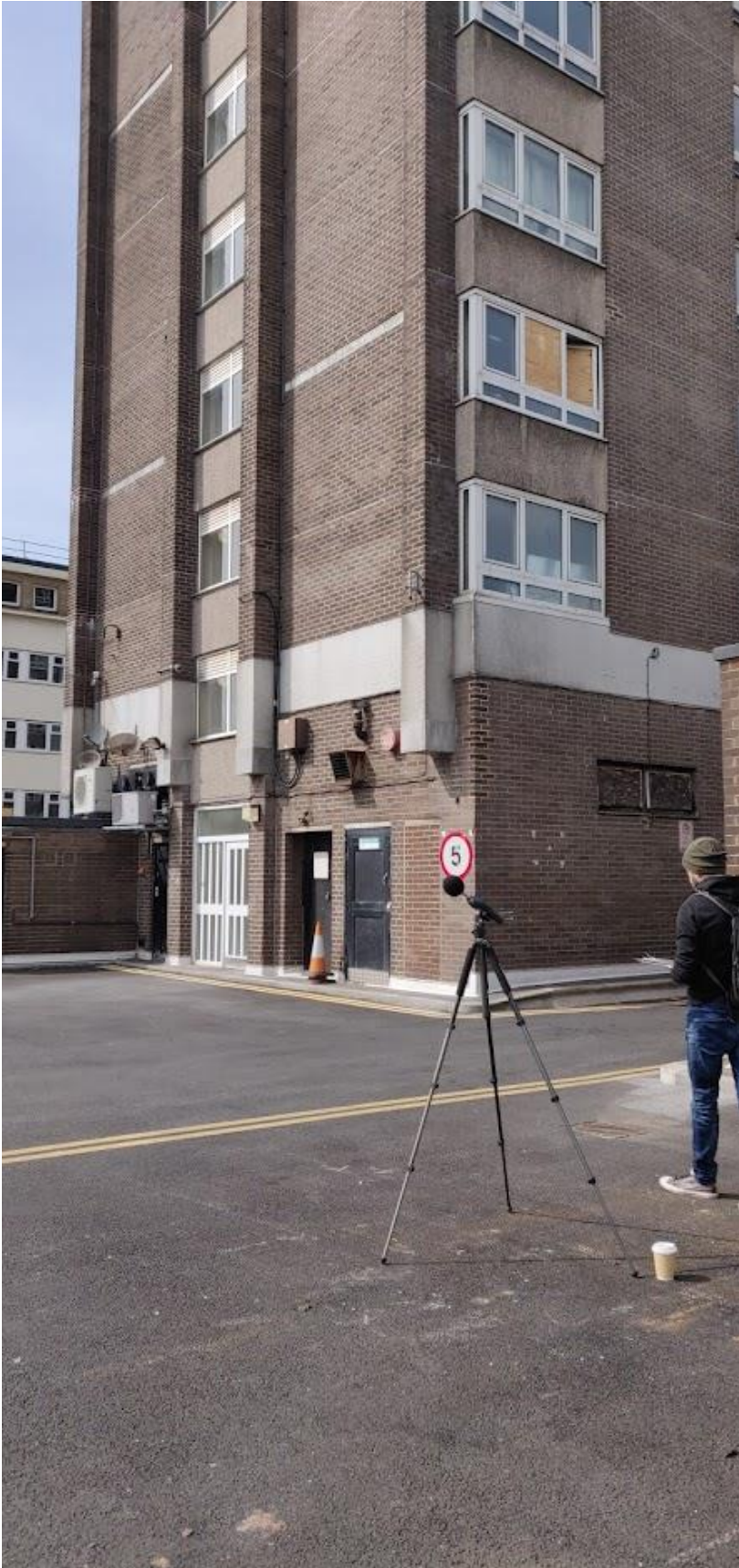
Figure B4: Location 2: Buxton House first floor (car park)
