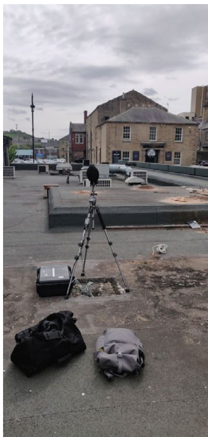
Figure B7: Market hall roof logger position
