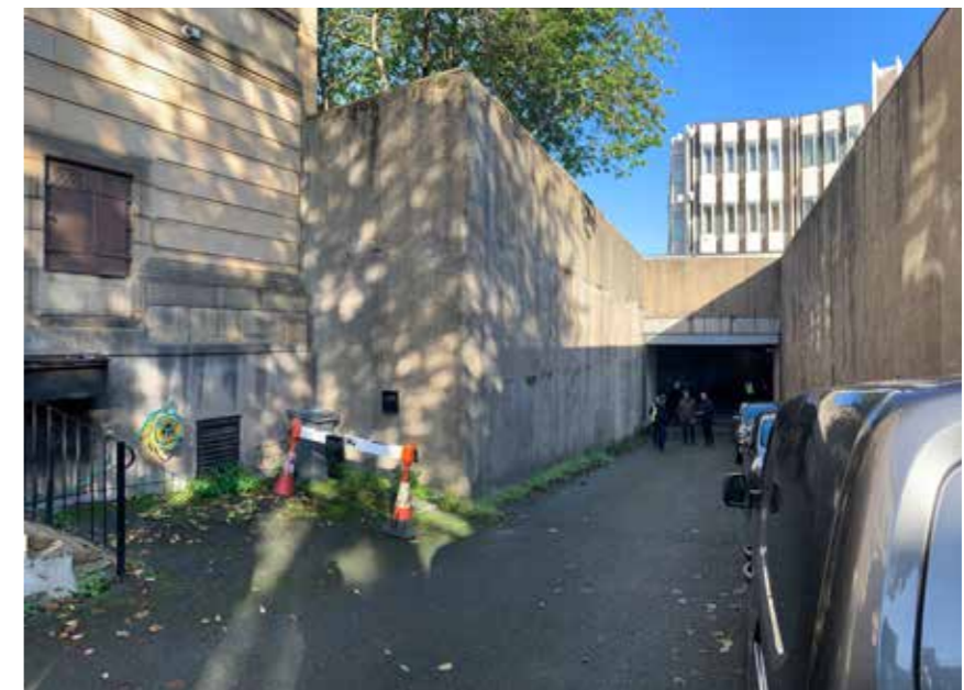
4.4.7 - Tunnel access below east elevation
