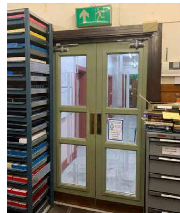
4.6.15 - Doors in Reference Archive (Rm.66)
