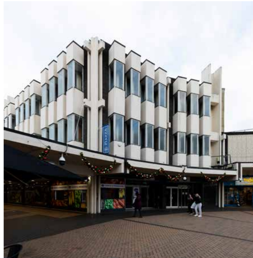
4.3.5 - Piazza Shopping Centre facing building's north aspect
