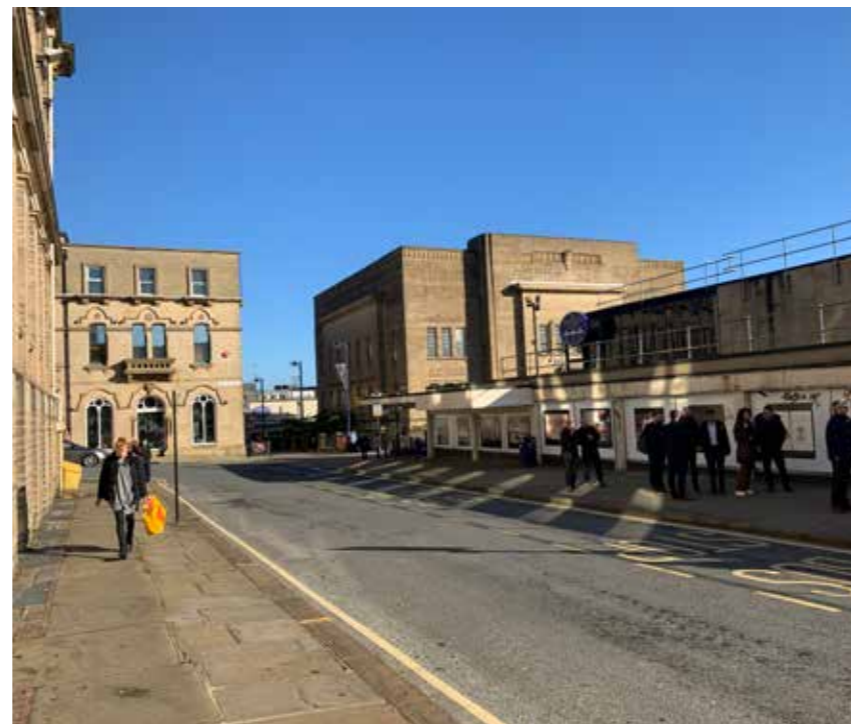
4.3.7 - View of building from Peel Street
