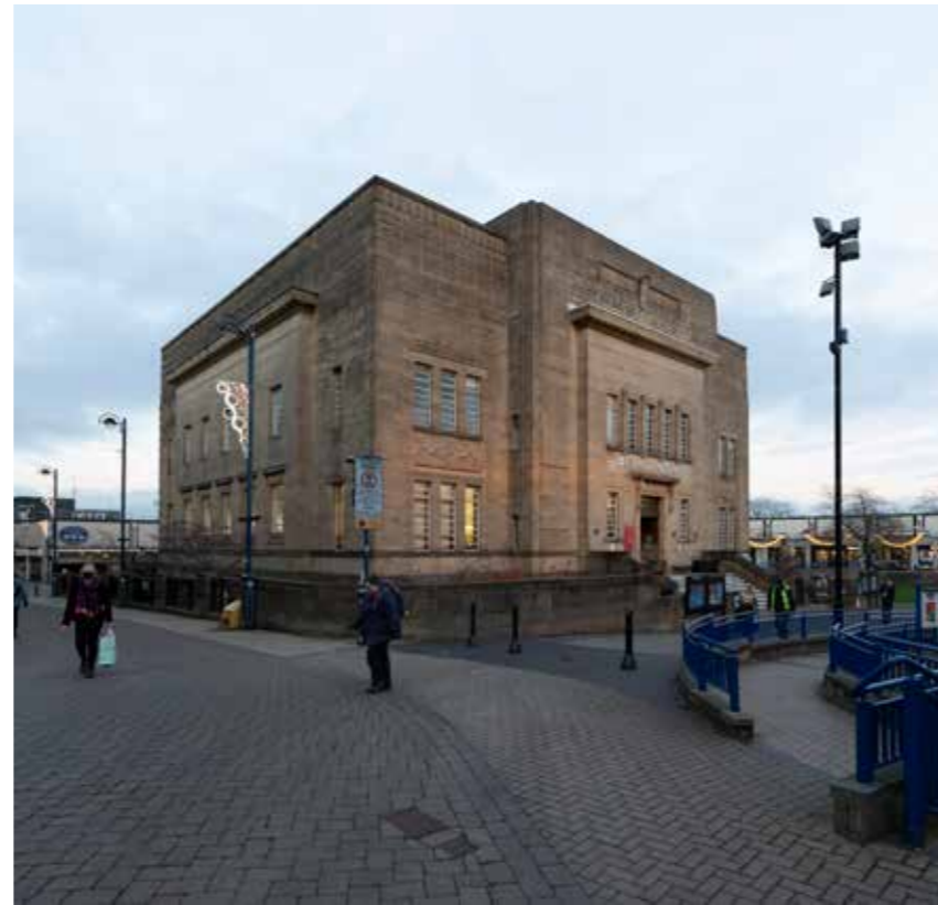
4.3.1 - Library and Art Gallery viewed from south-west
