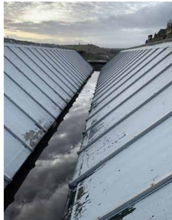
4.4.16 - Original lanterns to roof
