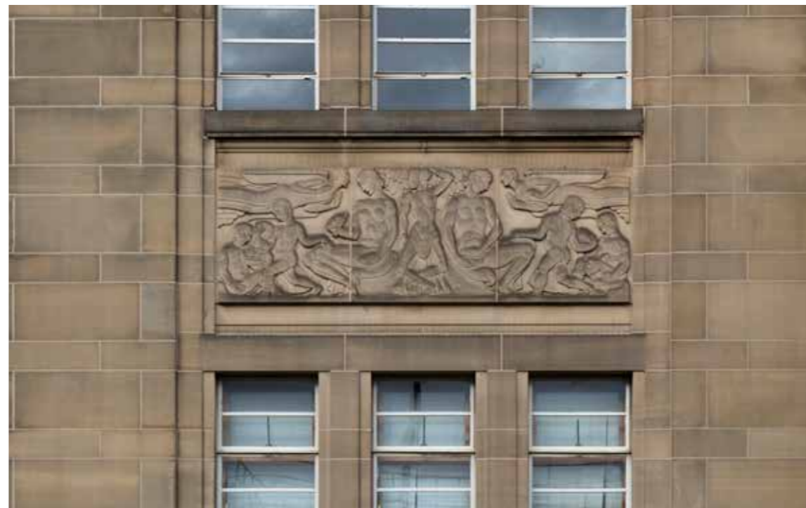
4.4.3 - Decorative panel on south elevation, James Woodford, 1939
