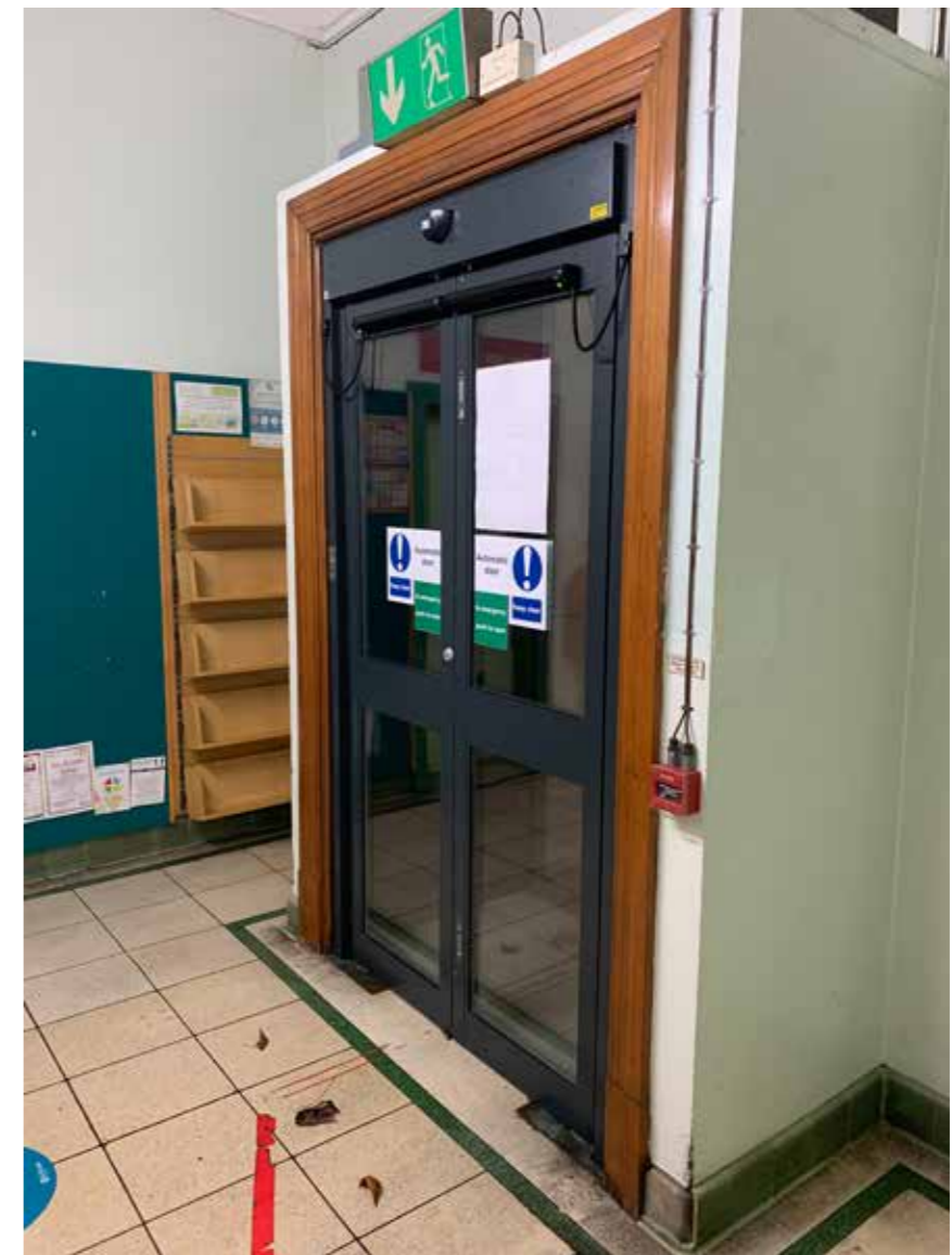
4.8.3 - East Entrance Lobby (Rm.28)
