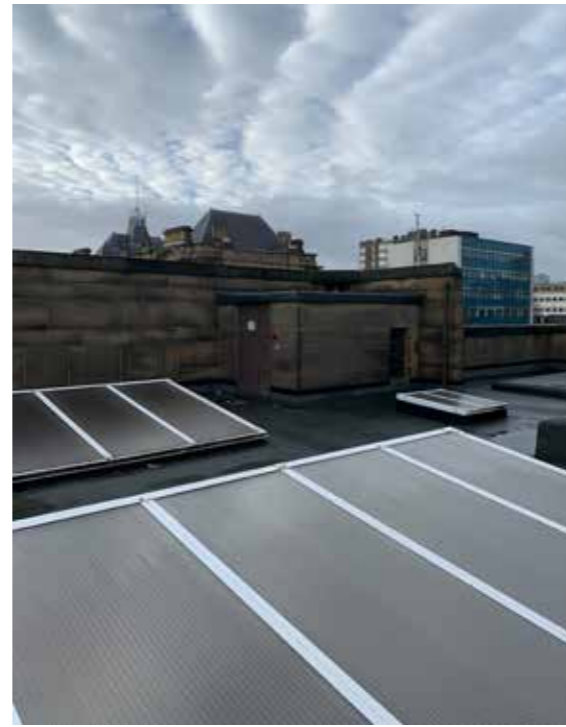
4.4.13 - Modern lanterns to roof
