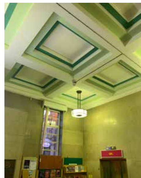
4.5.3 - Ceiling to Entrance Lobby / Reception (Rm.52)
