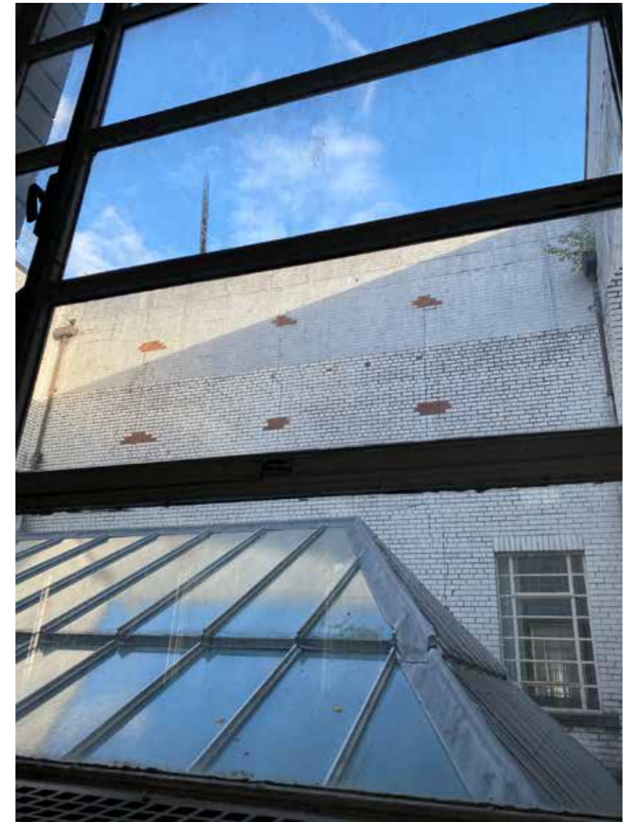
4.4.20 - Lightwell above atrium
