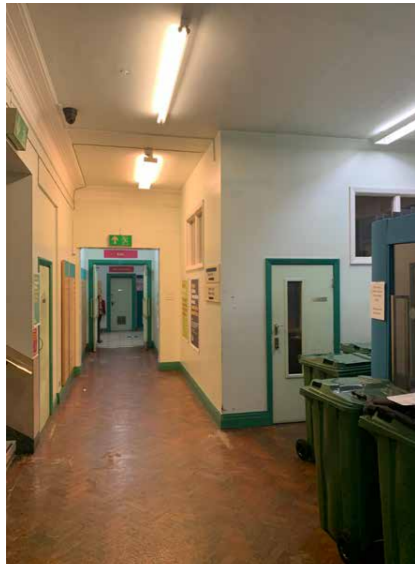
4.8.1 - Lower Ground Stair Lobby (Rm.24) with new room on right (Rm.26)
