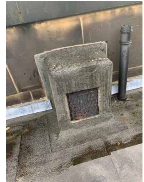
4.4.18 - Service access at roof
