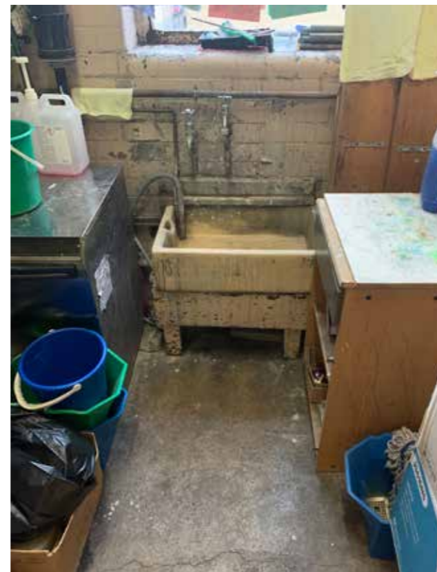
4.7.24 - Store / Service Room (Rm. 83)
