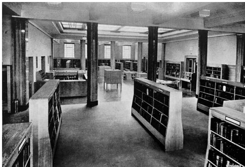
4.5.9 - Historic photograph of Main Lending Library (Rm.47)
