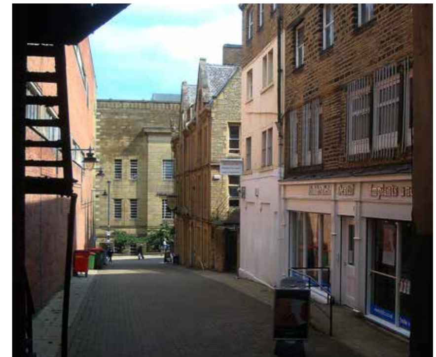
4.3.8 - View of west elevation from Albert Yard
