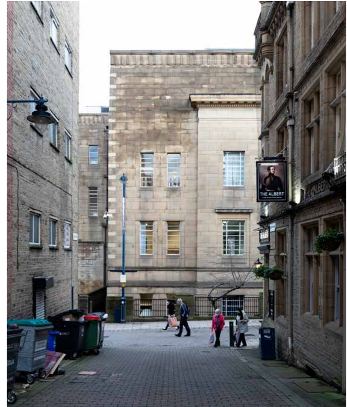
4.4.10 - East elevation from Albert Yard
