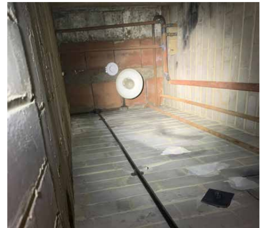
4.7.7 - Plant Space (Rm.89)
