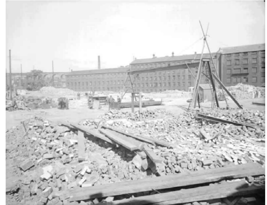
2.6.2.2 - Demolition of the Cloth Hall, 1930
