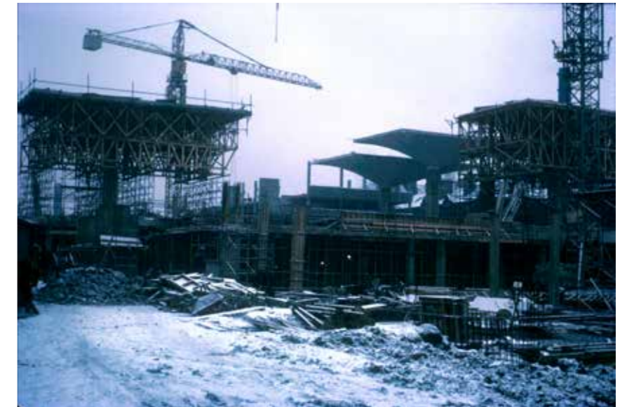
2.7.2.3 - Construction of the Murrayfield development, 1969
