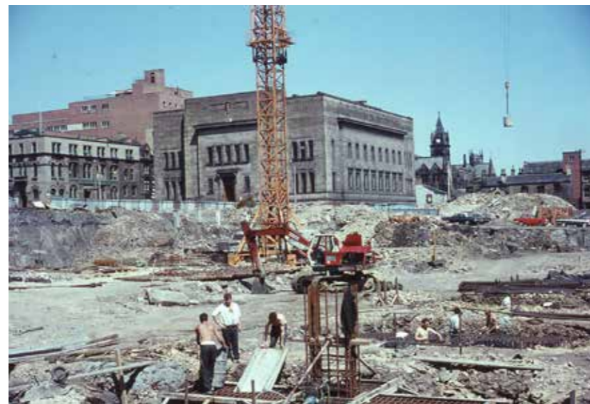
2.7.2.4 - Construction of the Murrayfield development, 1968
