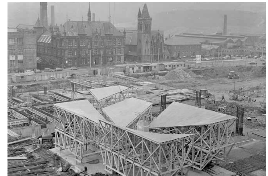
2.7.2.5 - Construction of the Murrayfield development, 1969
