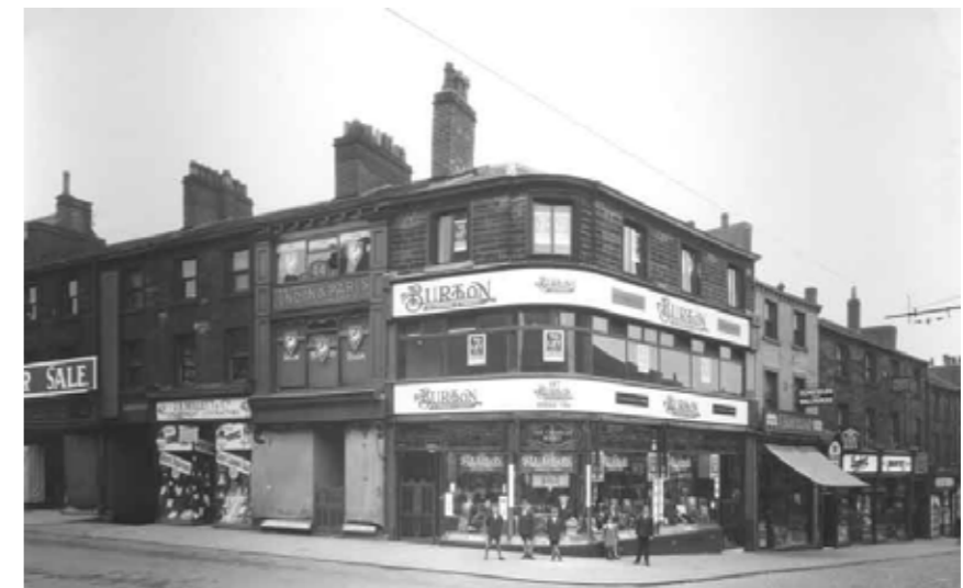
2.7.3.2 - Buildings at Kingsgate / Cross Church Street (now demolished), 1929
