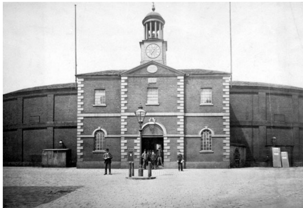
2.3.2.3 - Photo of the Cloth Hall (now demolished), c.post-1888
