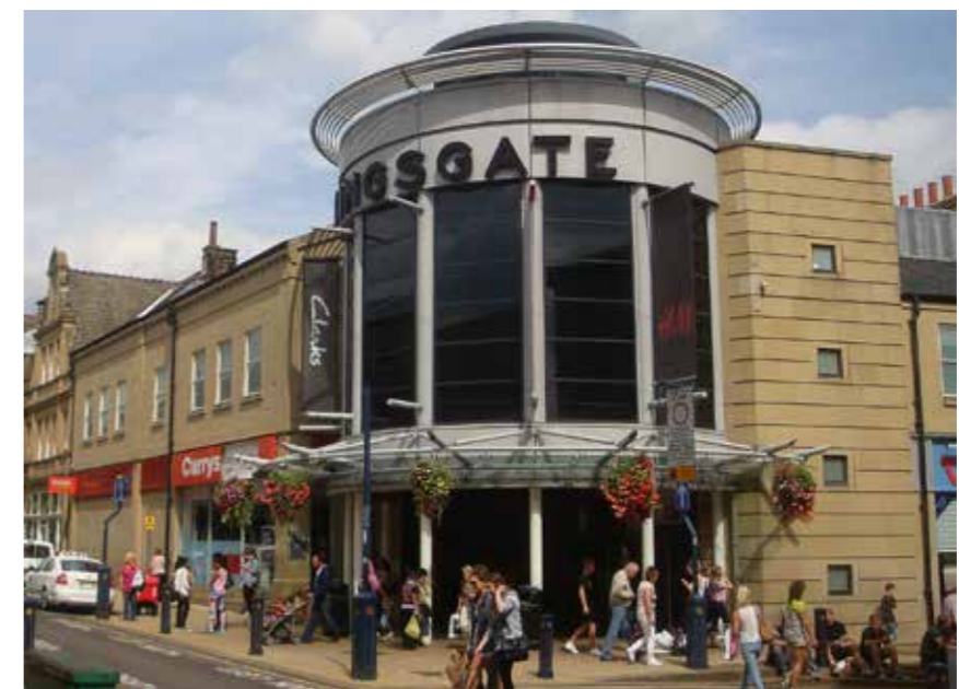
2.7.3.3 - Kingsgate Centre at Kingsgate / Cross Church Street, c.2010s
