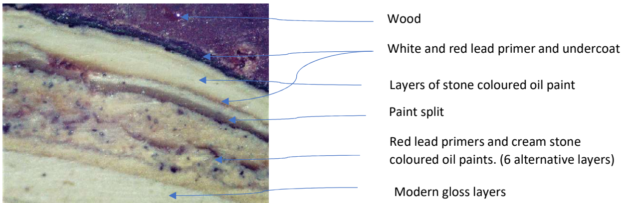
7. Outer window frame of middle bow sash on west elevation's first floor
