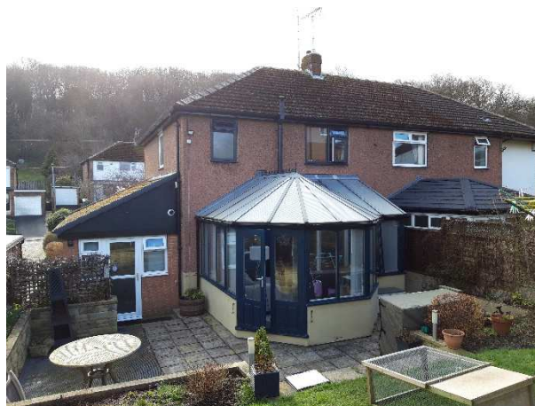
Photo 2: The building viewed from the rear garden.
