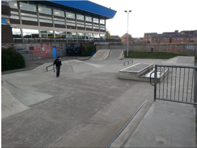
Original skatepark located at Spen Valley Swimming Pool. The old facility was demolished in 2019.
