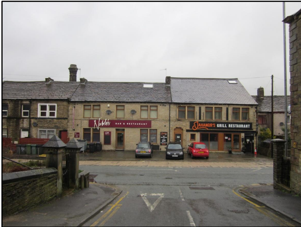
Photograph 2. A62 Manchester Road, existing residential dwellings and commercial premises to the North of the development site
