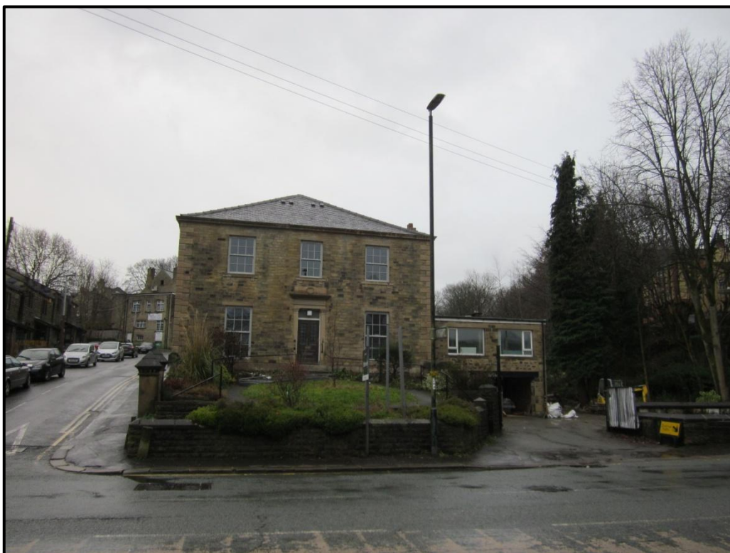
Photograph 1. Former Croft House Surgery and adjacent car port/office building
