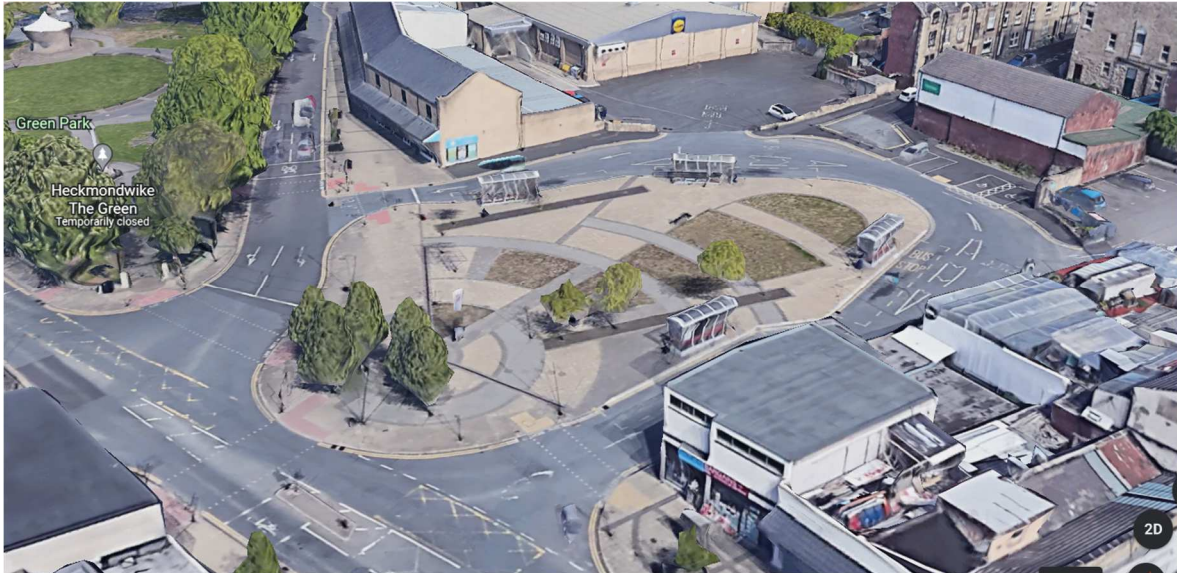
Aerial Google Earth image of the existing bus hub (taken from the southeast)
