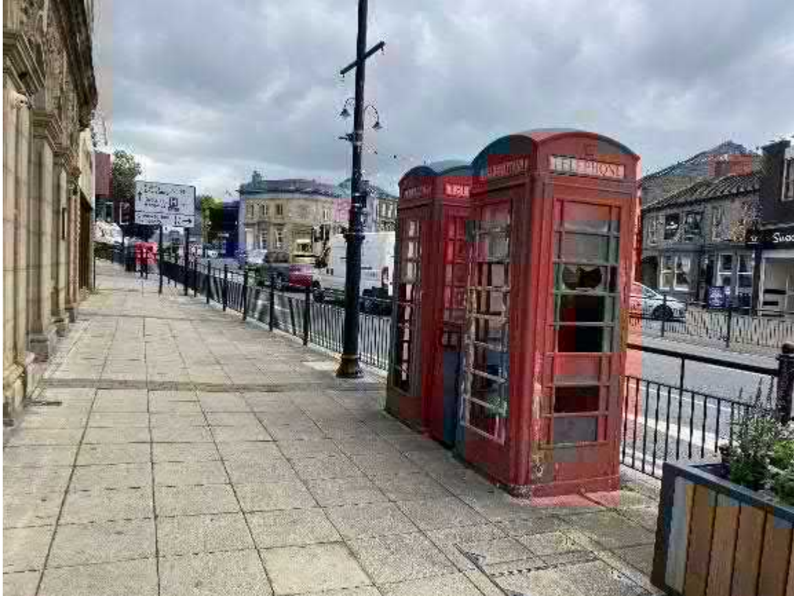
Image 6-2 - The Two K6 Telephone Kiosks outside the Midland Bank, looking east (HA03).
