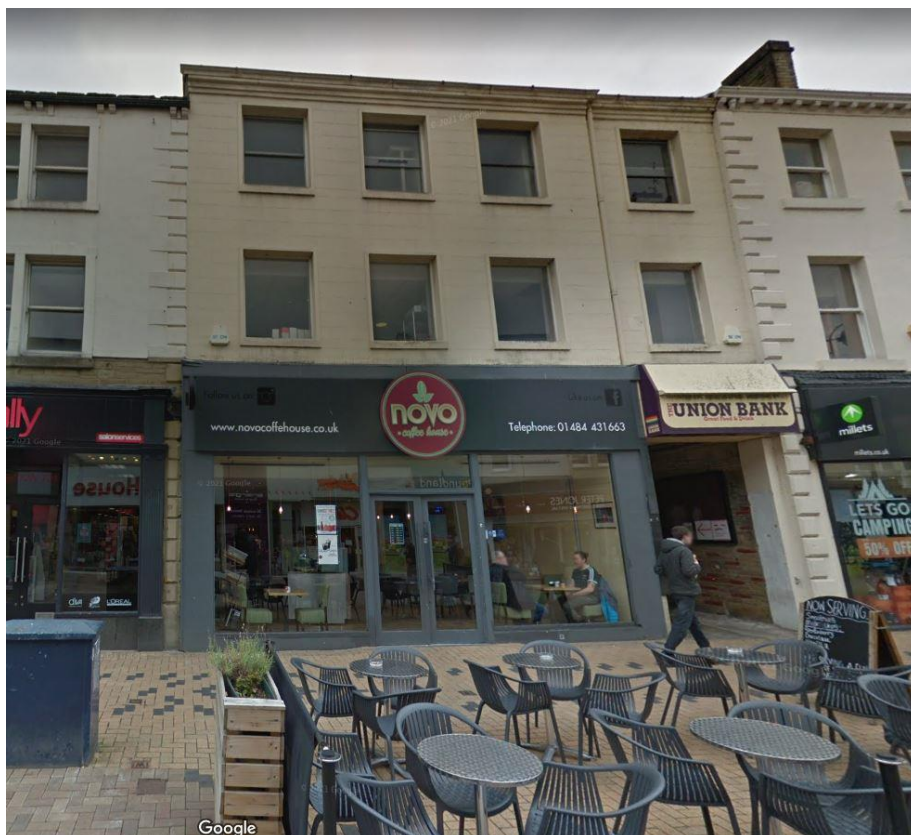
Photo showing the existing front façade of the property.
