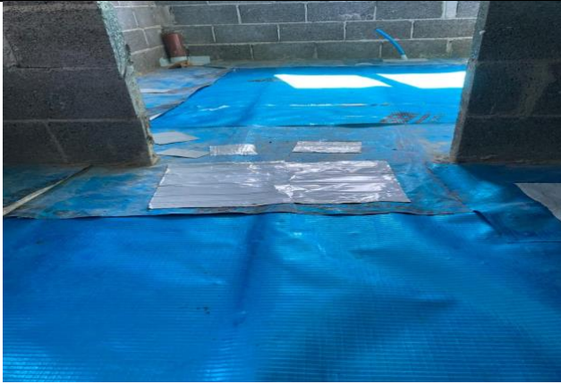
Patch Repair Entrance to Kitchen
