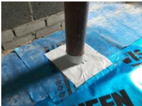
Sealed pipe using SAGM to Plot 5.
