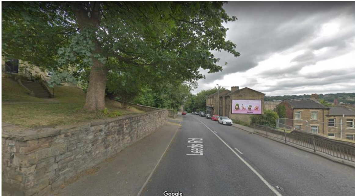
Fig 4: North East Facing Elevation of 37 Leeds Road, Dewsbury WF12 7BB with consented gable mounted 48s digital advertising display unit.
