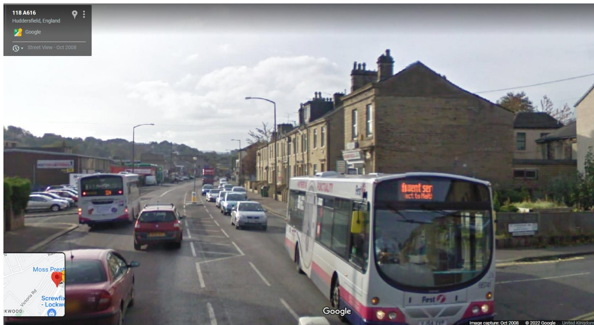
Fig 1: North Facing Elevation of 122 Lockwood Road, Huddersfield HD1 3QX in October 2008, which shows the lighter area of the gable where a 48 sheet billboard advertisement had been displayed.
