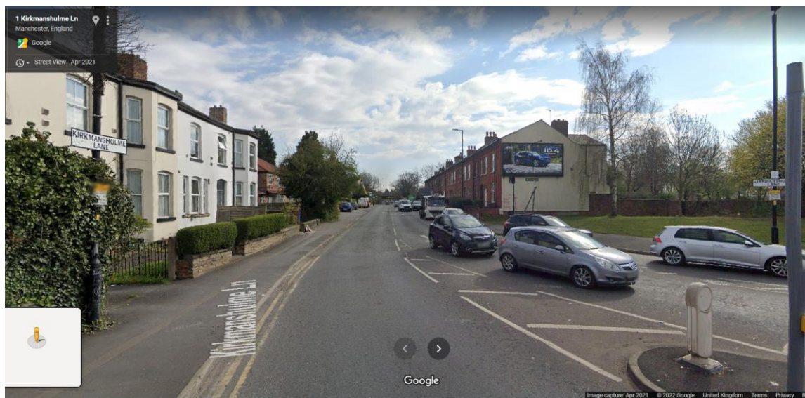
Fig 8: West Facing Elevation of Kirmanshulme Lane No 10, Manchester M12 4WA with consented gable mounted 48s digital advertising display unit.
