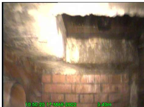
Photo: 4_10A 3.4m, Finish node type, manhole reference number: MH01
