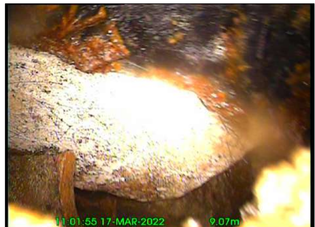
Photo: 5_12A 9.05m, Finish node type, manhole reference number: MH03
