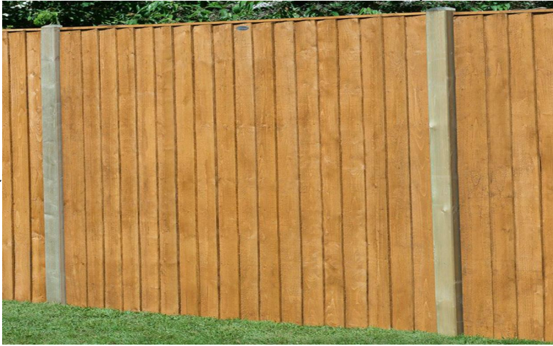
1.5m high Close-boarded Fencing
