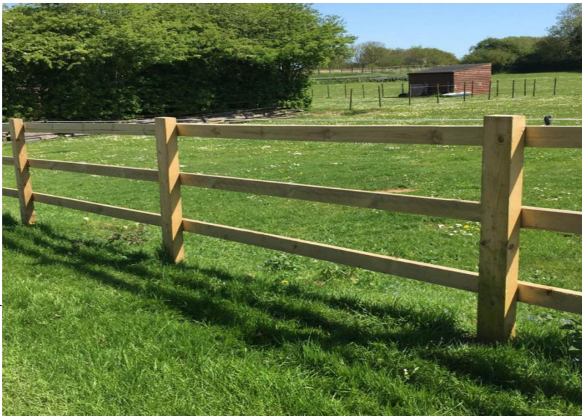
1.2m High Post + Rail Fencing
