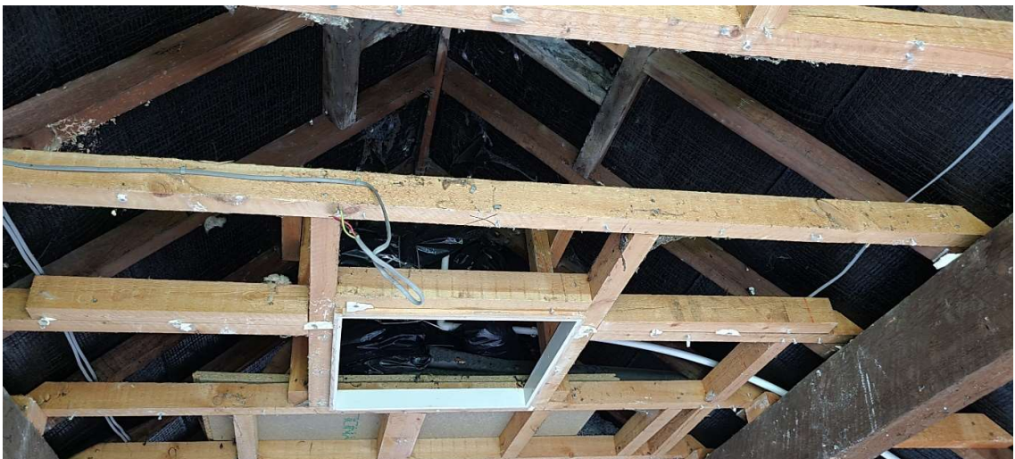
Plate 4. Inside of roof-space
