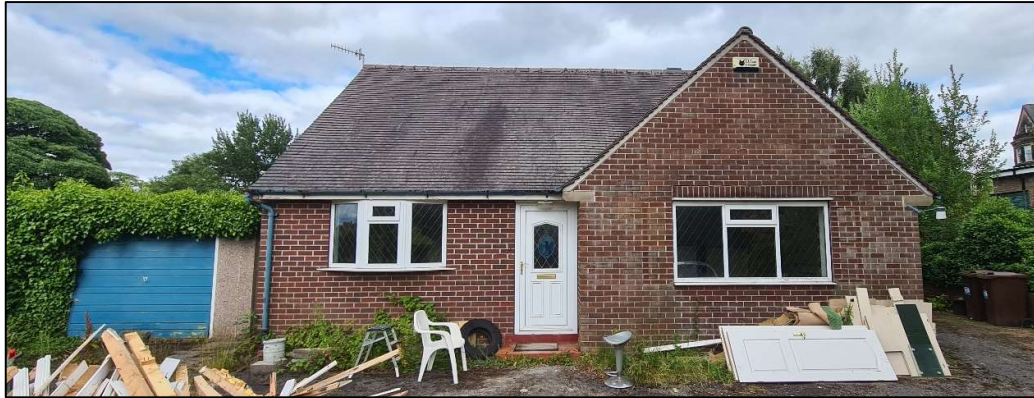
Plate 1. Front of the building (west elevation)
