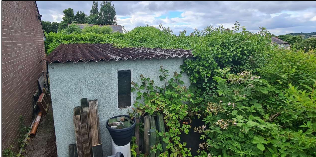
Plate 3. Rear of the garage including the roof
