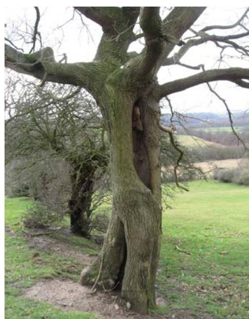
Photo 3 - Showing cavity openings in T26 oak.
