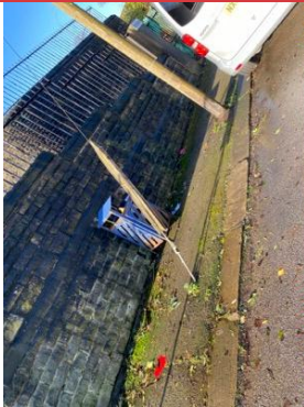
EXISTING RETAINING WALL Bottom Of Plane Street
