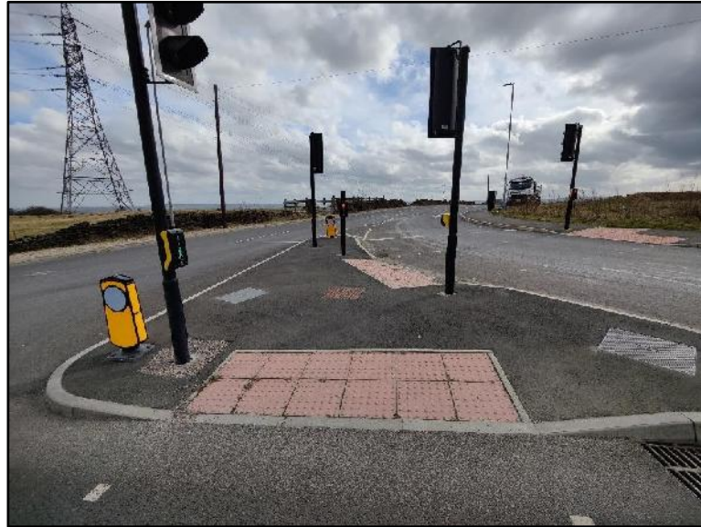
Photograph 2 - Crosland Road junction with Lindley Moor Road
