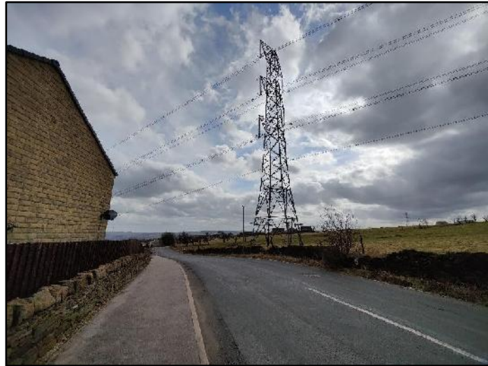
Photograph no. 3 – Weatherhill Road looking south east from the junction with the A643
