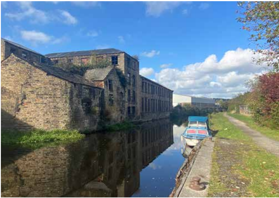
4. View north up the Broad canal
