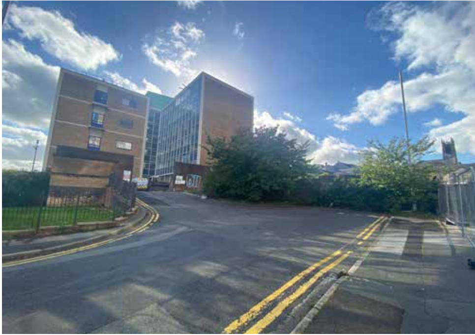
7. View south towards BT openreach building
