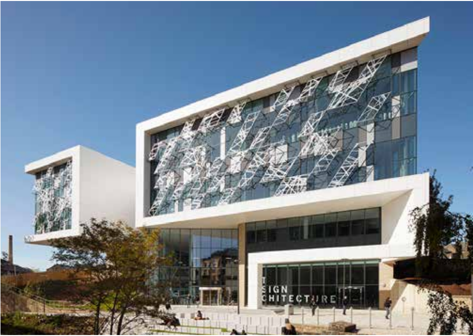
Fig 2.20.3 Barbara Hepworth Building, University of Huddersfield
