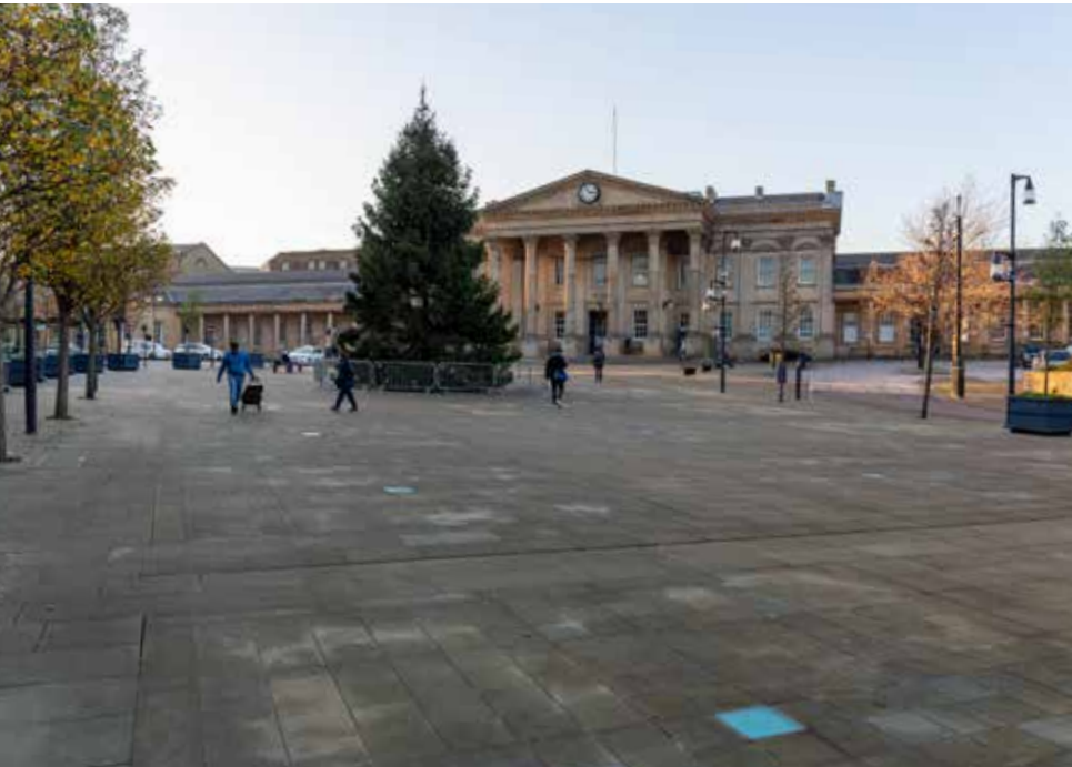
Fig 2.14.3 - St Georges Square and Huddersfield Railway Station
