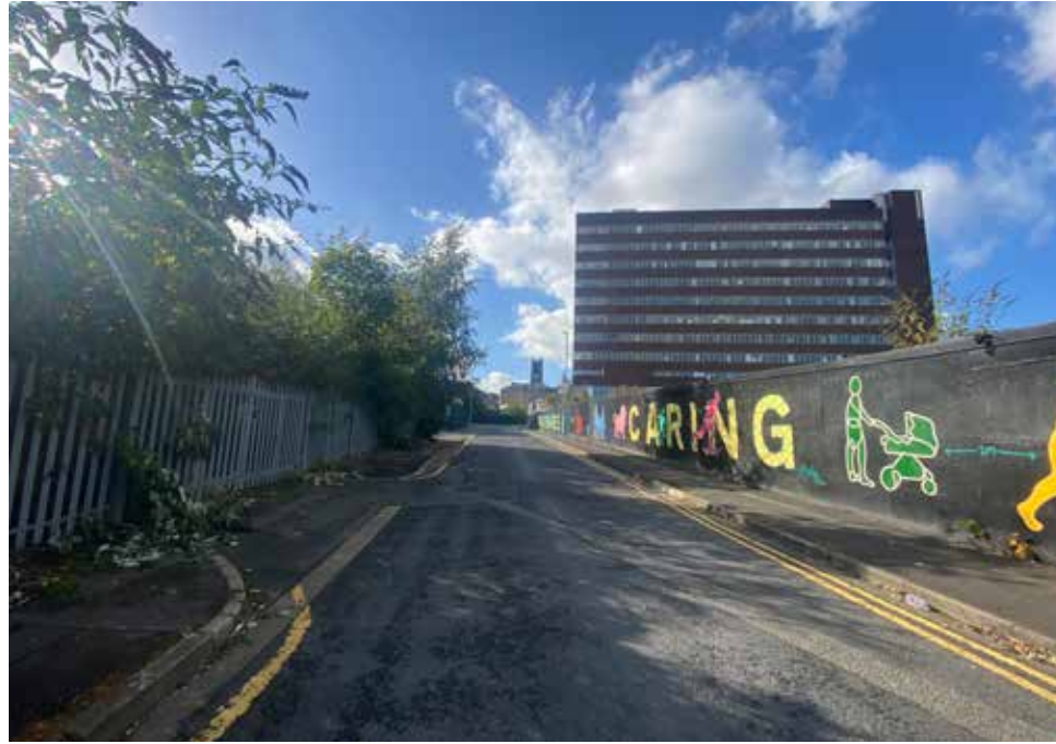
6. View south west up Old Leeds Rd
