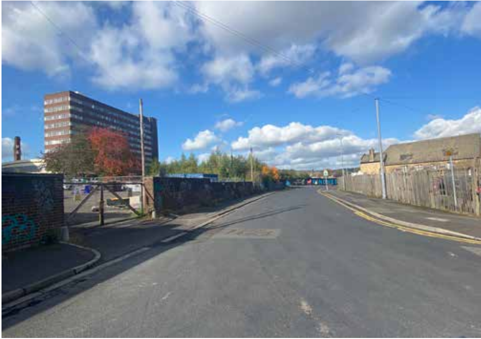
5. View north down Watergate
