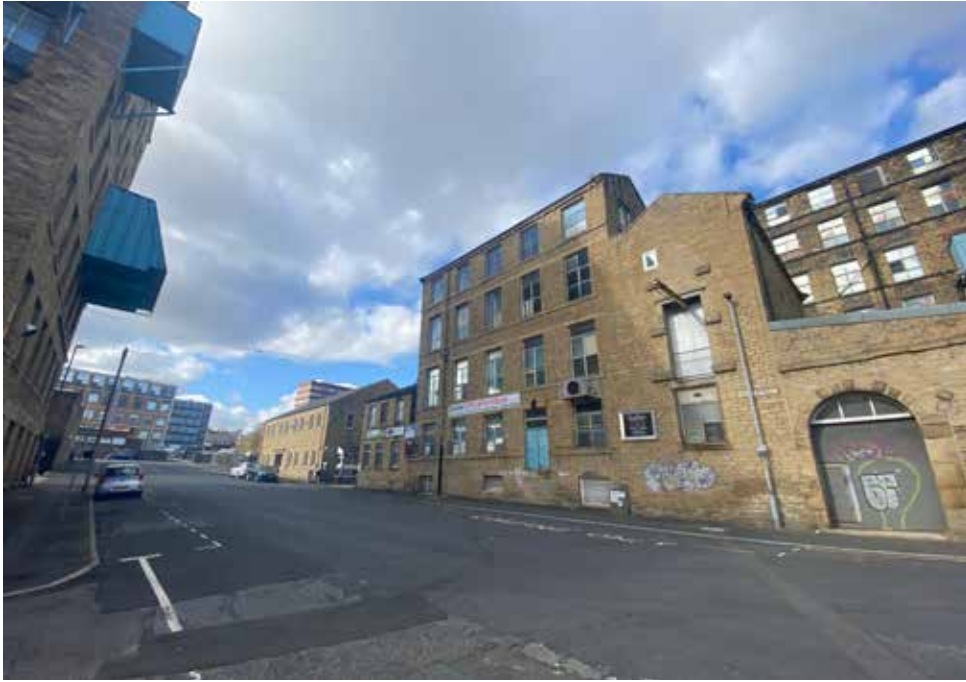
2. View north west down Quay St
