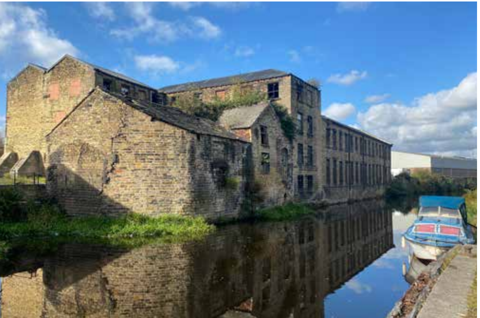
Fig 2.8.2 - Abandoned mill adjacent to the Southgate site.
