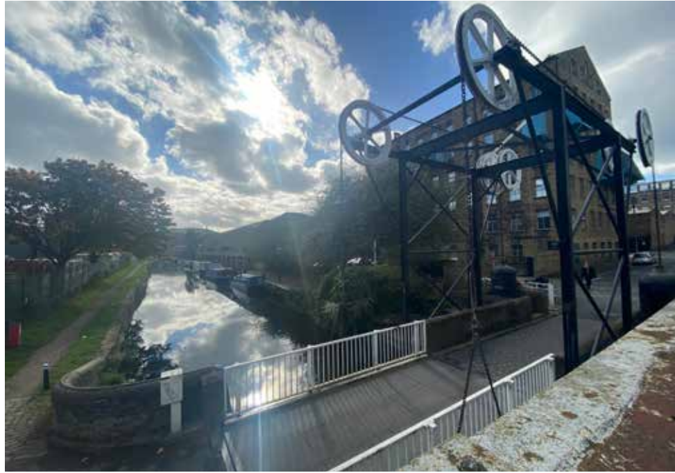
1. Canal bridge over the Broad Canal
