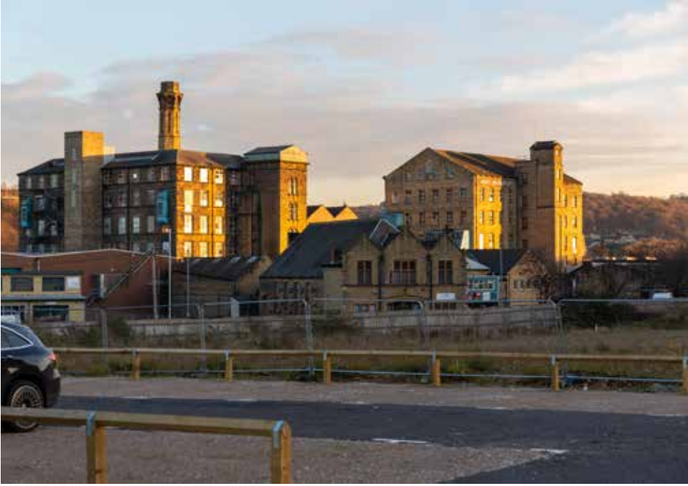
Fig 2.18.2 View east towards Broad Canal
