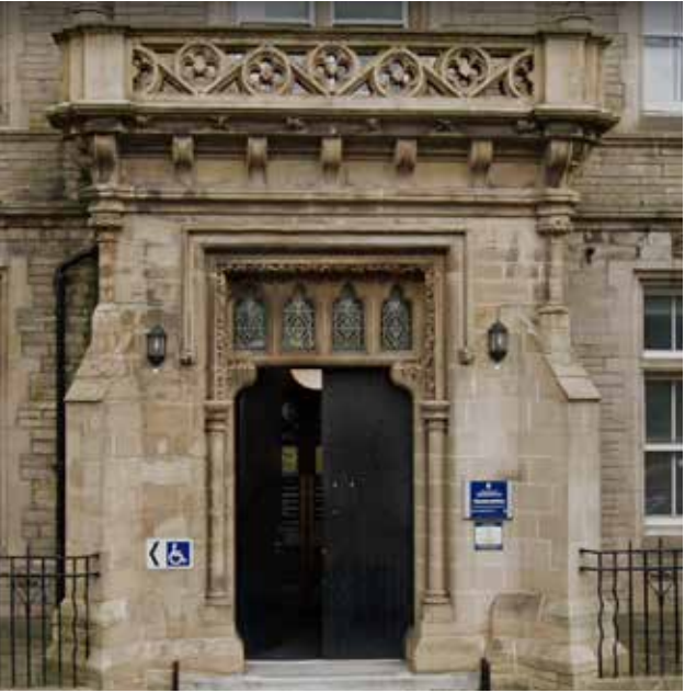
3. Ramsden Building, University of Huddersfield
